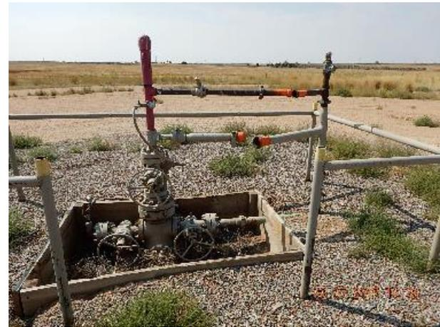
Photo 2: Disconnected wellhead and riser.
