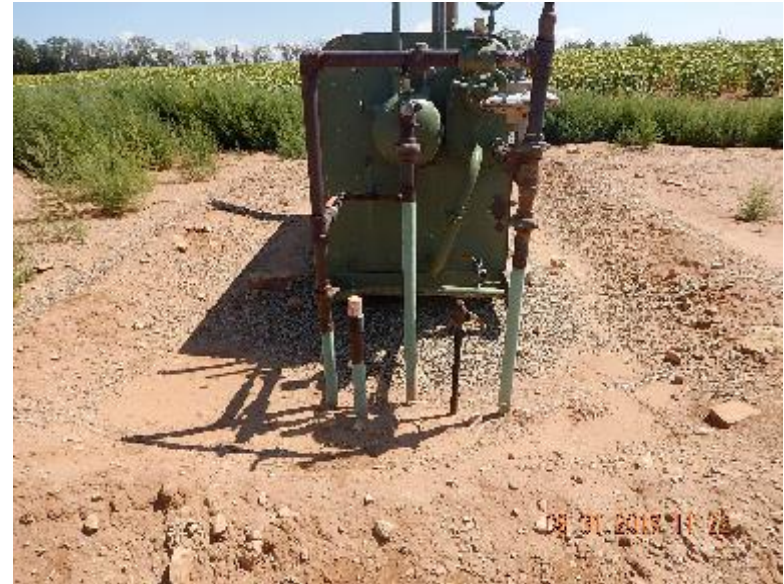
Photo 2: Disconnected risers at separator.
