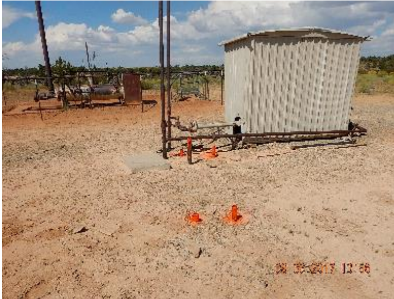
Photo 3: Risers (5) beside gas meter shed.
