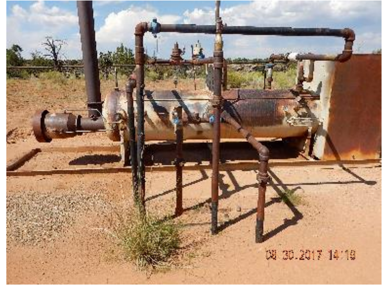
Photo 6: Flowline risers at separator.
