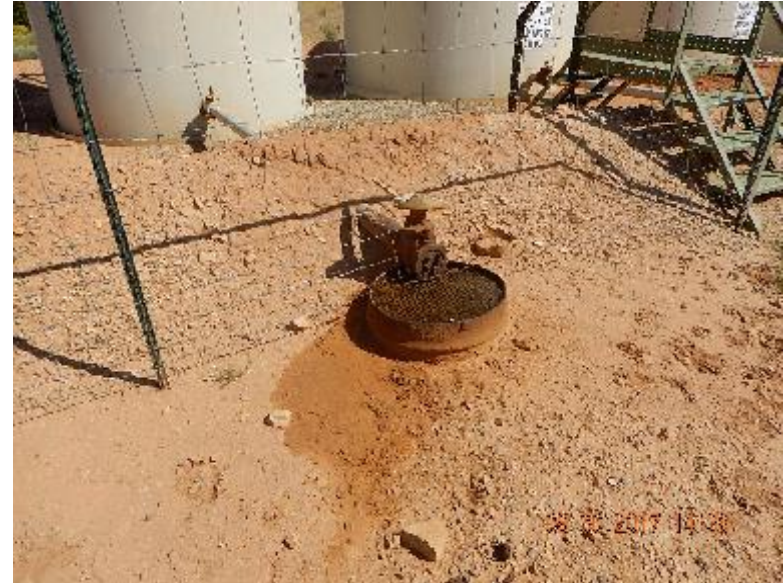
Photo 12: Water tank load out spill prevention full and impacted soil from overflow.
