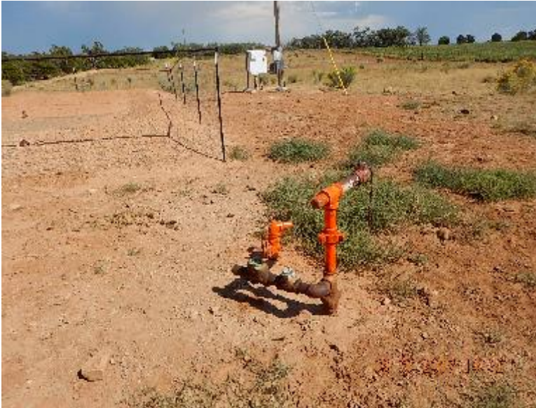
Photo 7: Risers outside production tank battery fencing.
