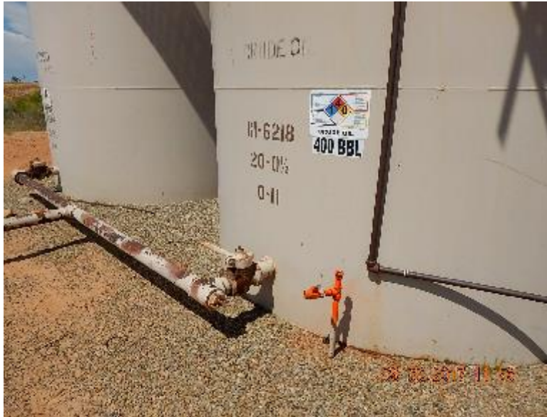
Photo 7: Riser in production tank battery.
