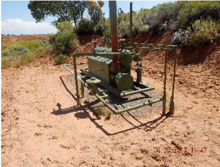
Photo 3: Separator and risers.
