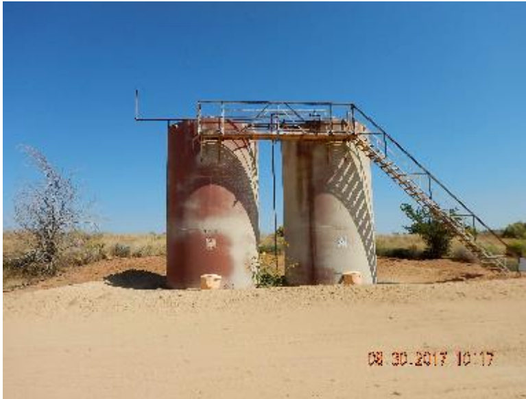
Photo 3: Tank battery.
