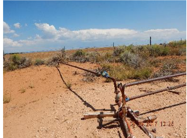
Photo 8: Above ground steel and black poly line on E side of location leaving location.
