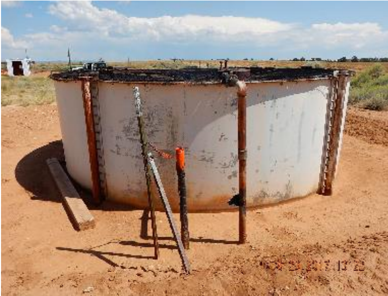
Photo 3: Riser at produced water open top tank.
