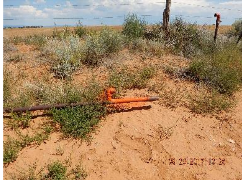
Photo 10: Closer view of open ended line and riser behind gas meter run house.
