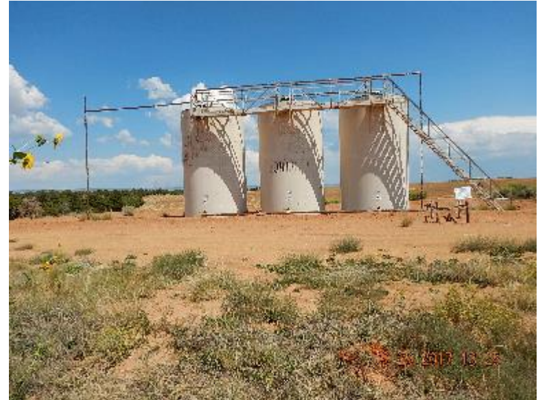
Photo 6: Production tank battery.
