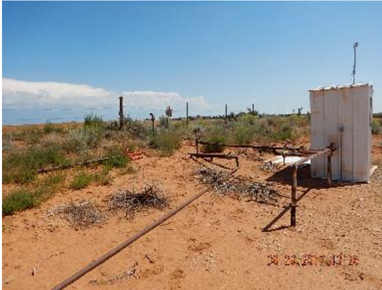
Photo 9: Open ended line and riser behind gas meter run house.
