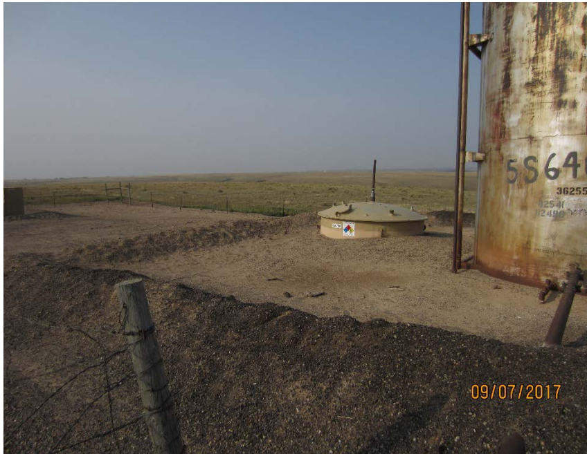
Photo #5 – Shallow/eroded earthen berm south of produced water vault.
