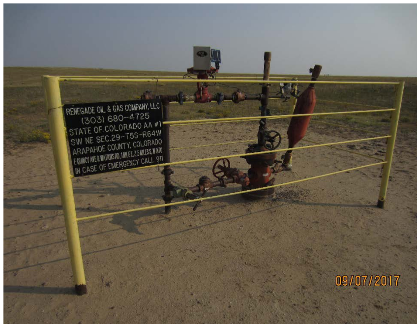
Photo #1 – Wellhead and sign.
