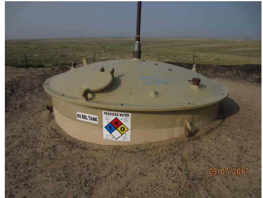
Photo #4 – Label and placard on produced water vault.
