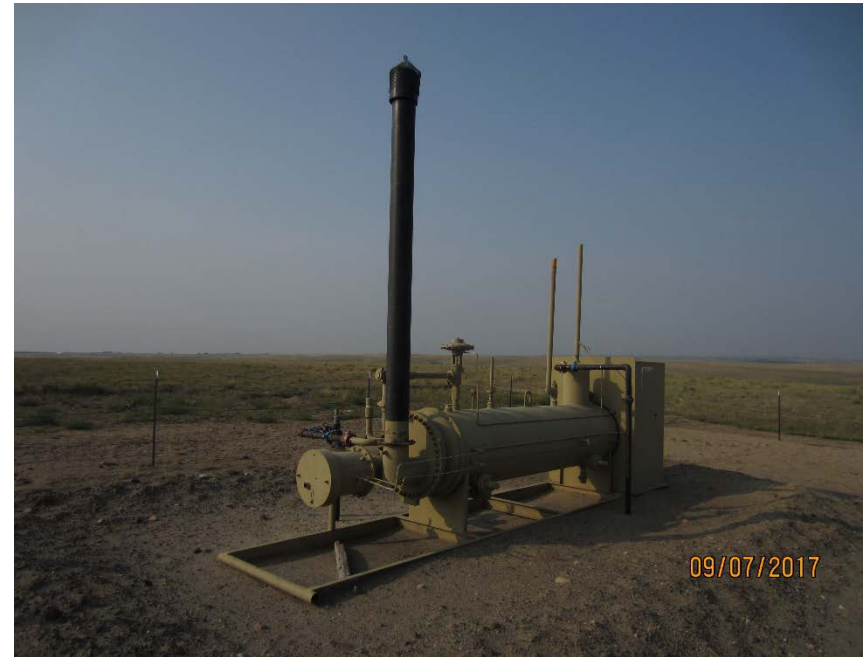
Photo #6 – Horizontal separator south of tank battery.
