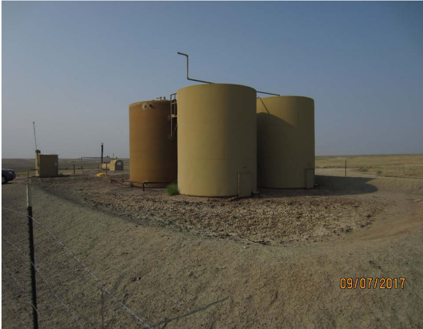
Photo #7 – View of tank battery from NE corner. Note that berm is shallow due to erosion.
