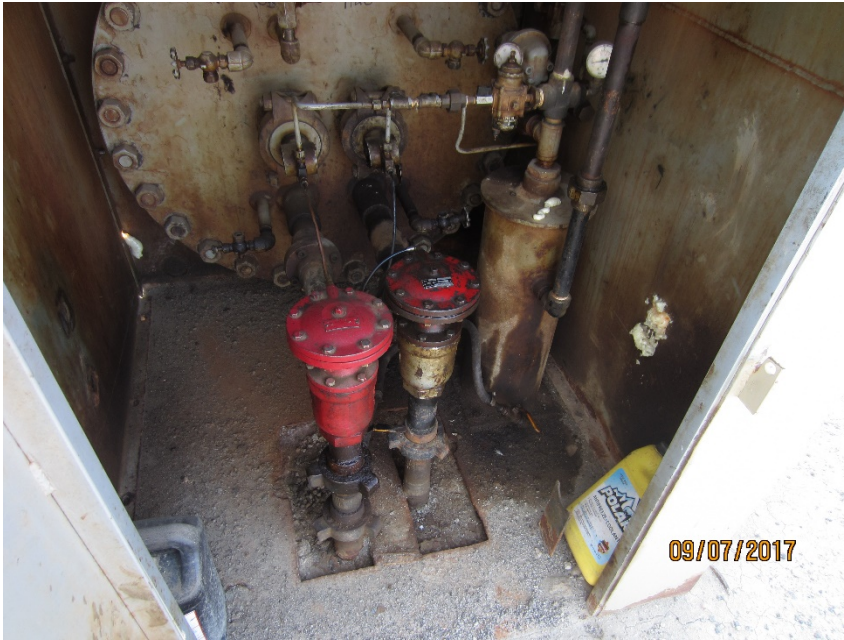
Photo #11 – Localized, oil-stained soil and equipment on north side of separator.
