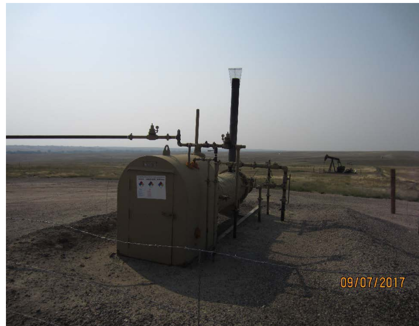
Photo #10 – Heated horizontal separator with barbed wire fence and bird protection.
