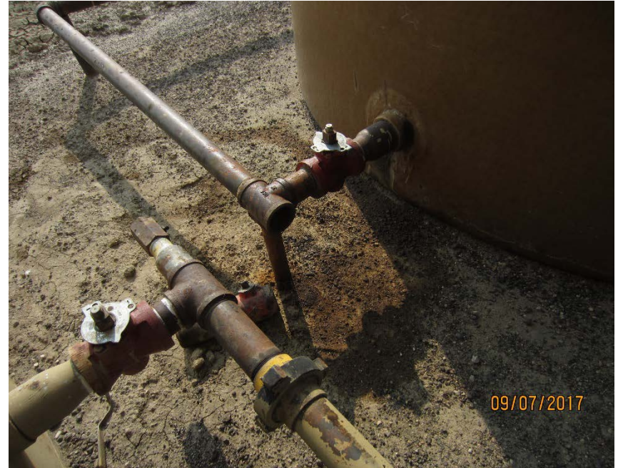
Photo #8 – Localized, oil-stained soil beneath valve on north side of produced water AST. Note uncapped pipe in center of photo.
