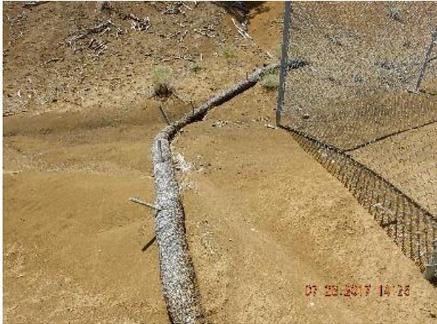
**Photo 7: Previous inspection waddle and sediment flow in SW corner.**
