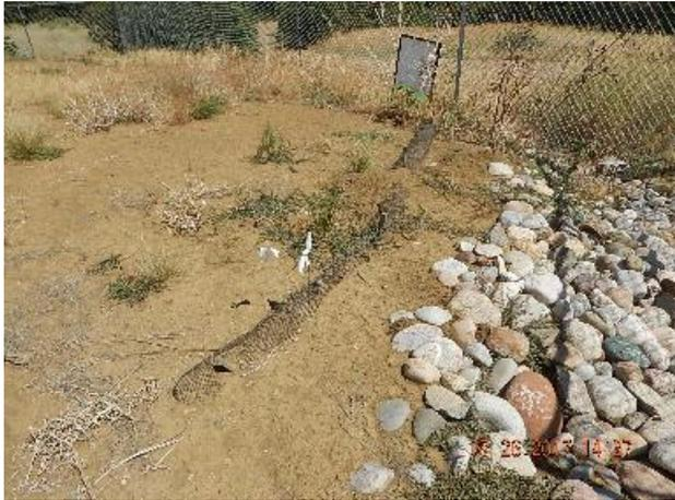
**Photo 11: Previous inspection waddle and sediment flow at location entrance.**
