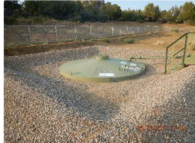
**Photo 4: Repaired berms and base of containment.**
