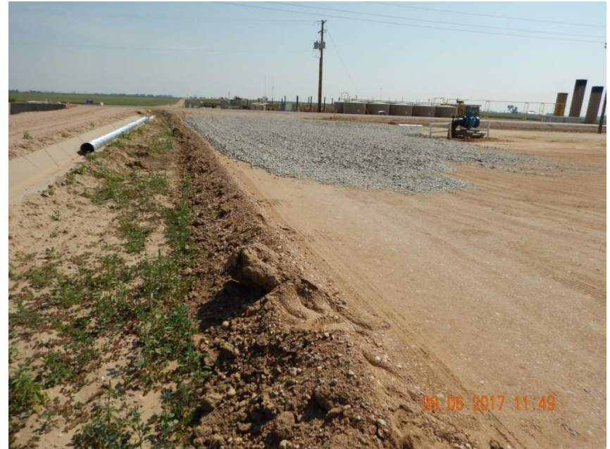
Photo 10. Photo taken from the entrance of the production facility, facing East. Tracking pad device installed at location. Unconsolidated berm observed along portions of the northern production facility.
