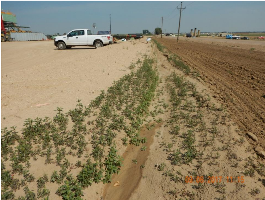
Photo 3. Photo taken from the southeast well pad location, facing North. Ditch and berm BMP installed around the perimeter of the well pad location.
