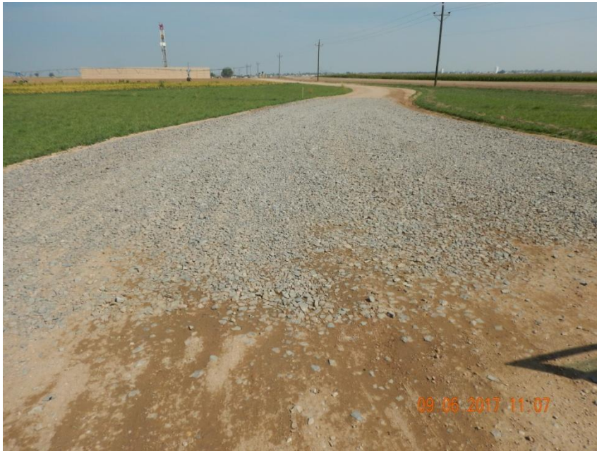
Photo 1. Photo taken from the entrance of the well pad location, facing North. Tracking pad device installed at location.
