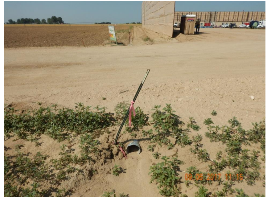
Photo 2. Photo taken from the southeast well pad location, facing West. Ditch and berm BMP installed around the perimeter of the well pad location.
