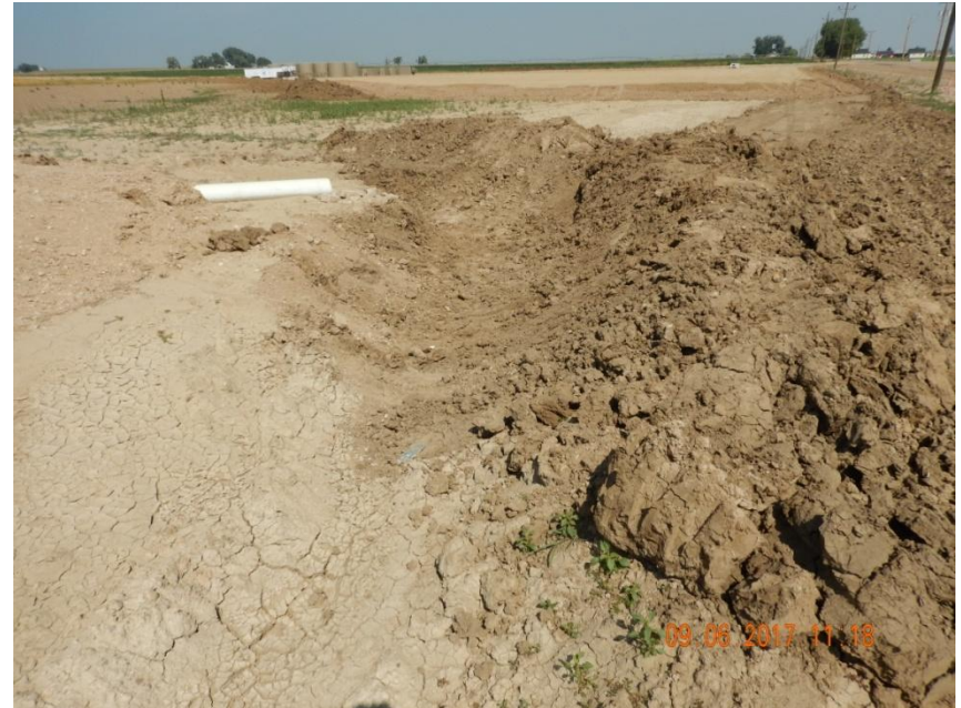
Photo 4. Photo taken from the northeast well pad location, facing North. Sediment trap embankment berms have not been compacted and still needs a stabilized outlet structure.
