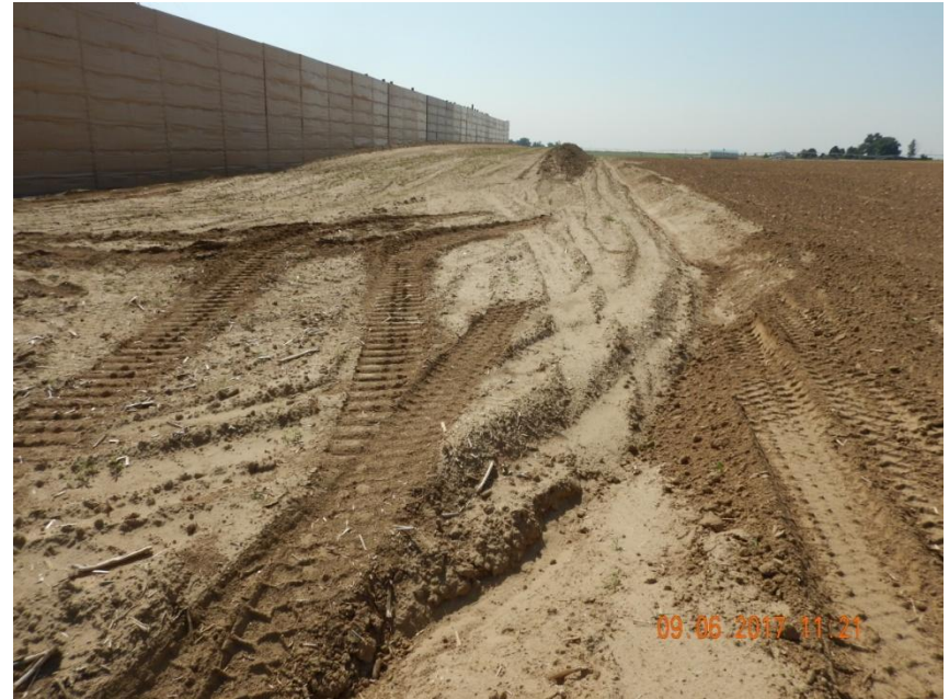
Photo 6. Photo taken from the northwest well pad location, facing South. Ditch and berm BMP installed around the perimeter of the well pad location. Also, photo illustrates topsoil stockpile stored along the west perimeter of the location.
