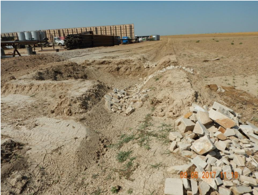
Photo 5. Photo taken from the northeast well pad location, facing West. Sediment trap installed with a stabilized outlet structure.
