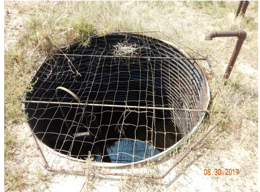
Photo #10 – Tinhorn skim pit with fluid remaining. Note: flowline risers in and outside of pit and damaged mesh (toward top of photo).
