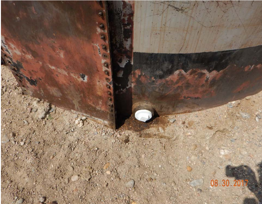
Photo #5 – Localized, stained soil beneath east crude oil AST, as indicated in previous FIR.
