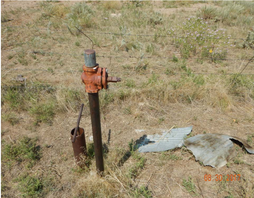
Photo #11 – Abandoned 2" flowline riser and 4" riser for valve control located NW of tinhorn.
