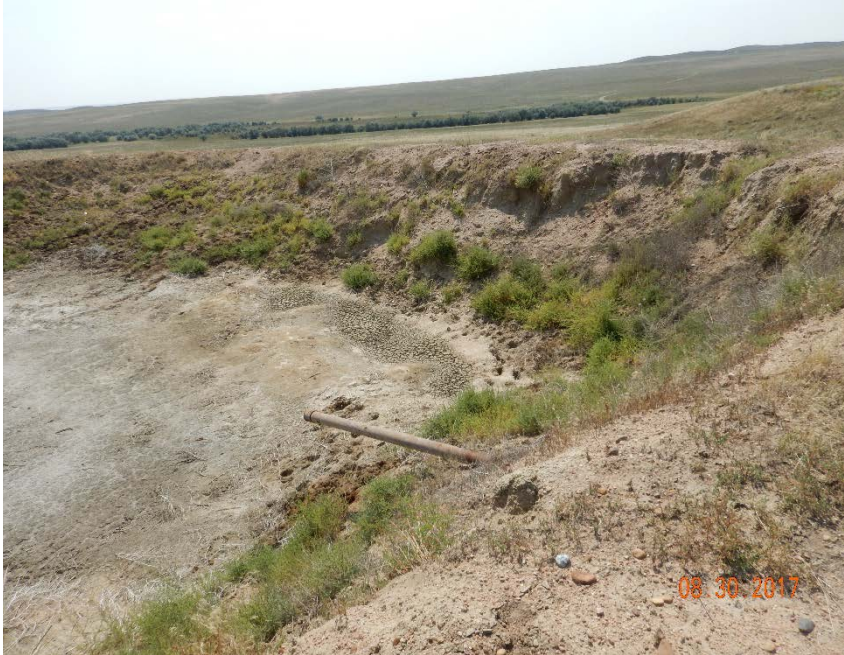
Photo #13 – View of produced water pit from tinhorn (looking SW). Note: localized, oil-stained waste underlying inlet from tinhorn.
