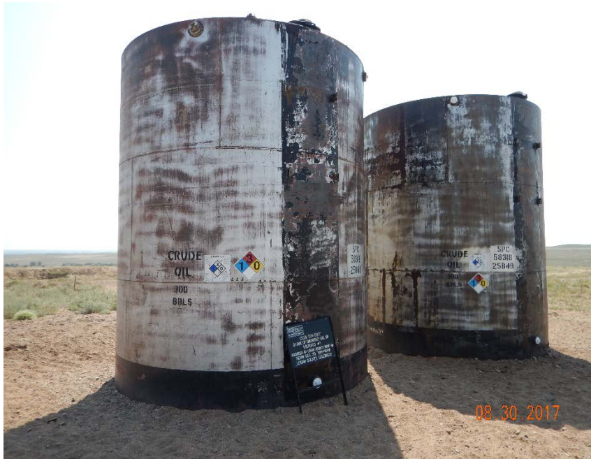
Photo #3 – Crude oil ASTs lacking earthen berm.
