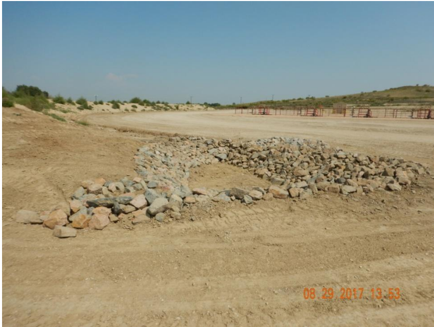
Photo 3. Photo taken from the northwestern facility, facing East. Appears the Operator has installed a sediment trap in conjunction with a ditch- see Photo 4.
