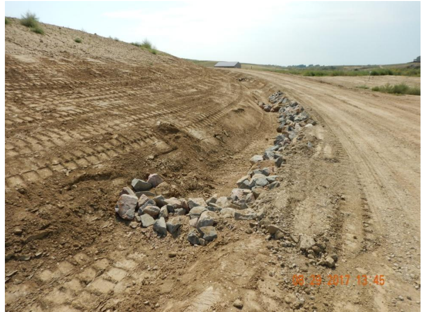
Photo 4. Photo taken north of the previous sediment trap, facing South. Operator has installed a ditch, armored with rock along portions, as well as check dams. Stormwater runoff appears to be directed to the sediment basin along the northeastern facility- see Photo 5.
