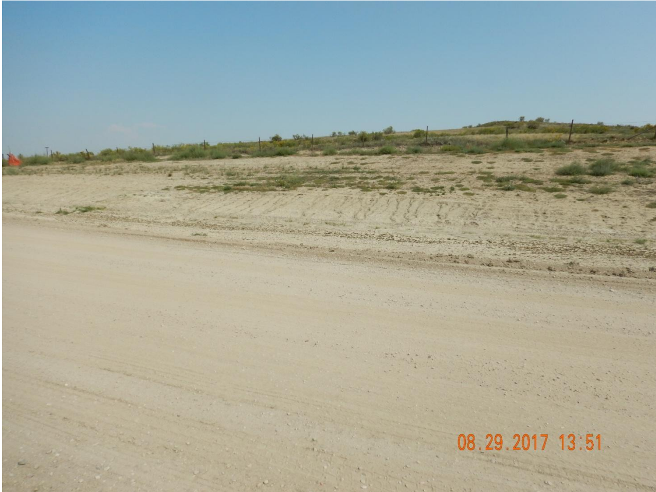
Photo 8. Photo taken from the eastern location, facing East. Does not appear the Operator has repaired rill erosion along the entire eastern cut slope.
