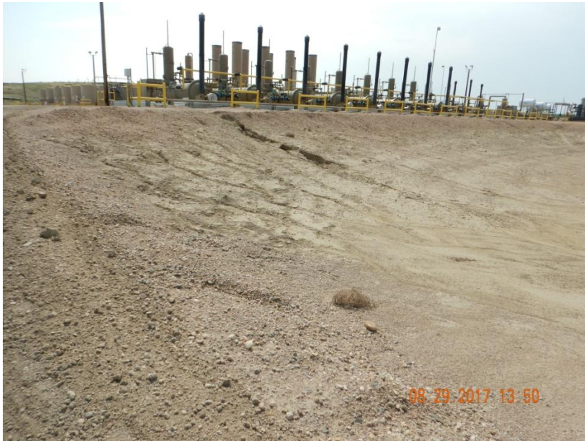
Photo 9. Photo taken from the east-central location, facing Southwest. Does not appear the Operator has repaired rill/gully erosion along the fill slope.
