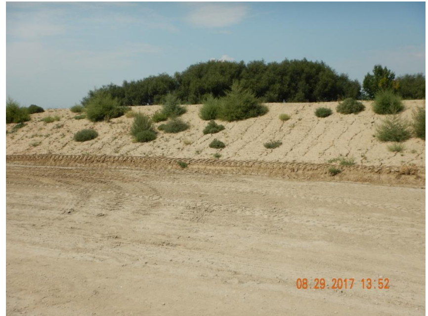
Photo 10. Photo taken from the central location, facing Northwest. Does not appear the Operator has repaired rill erosion along the soil stockpile.
