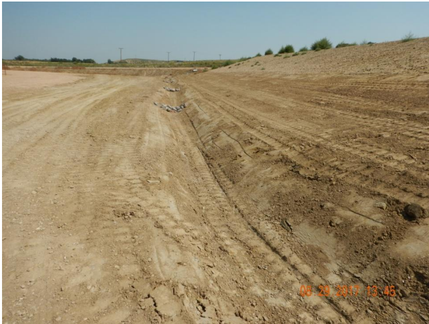
Photo 5. Photo taken from the previous Photo 4 location, facing East. Ditch has been installed that appears to be directed to the sediment basin along the northeastern facility.
