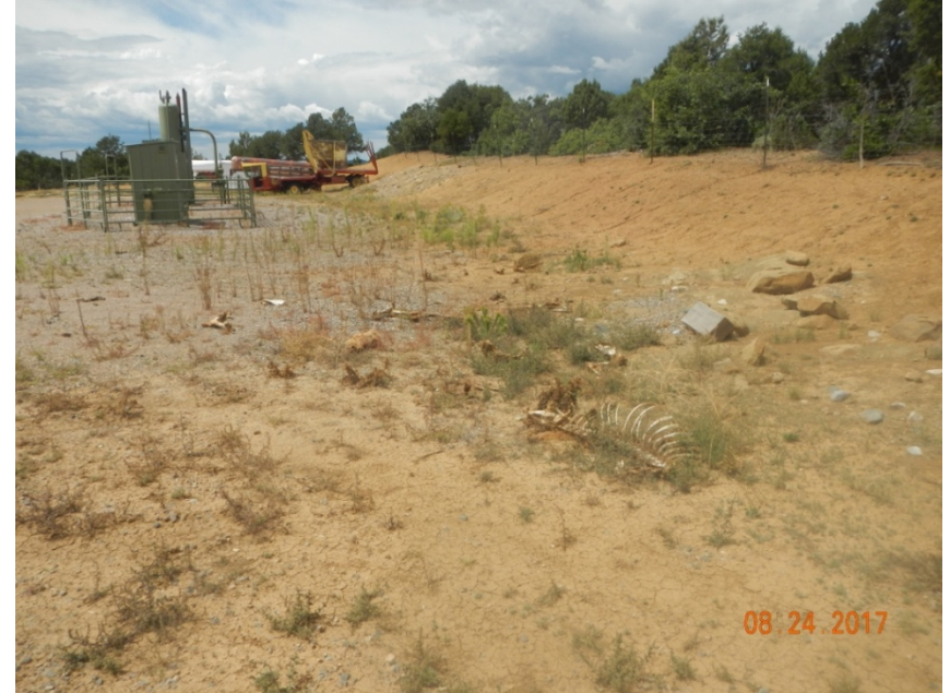
Photo 4: View of the northern portion of the project area from the northeastern corner facing westward. Exposed cut-slope is not stabilized.
