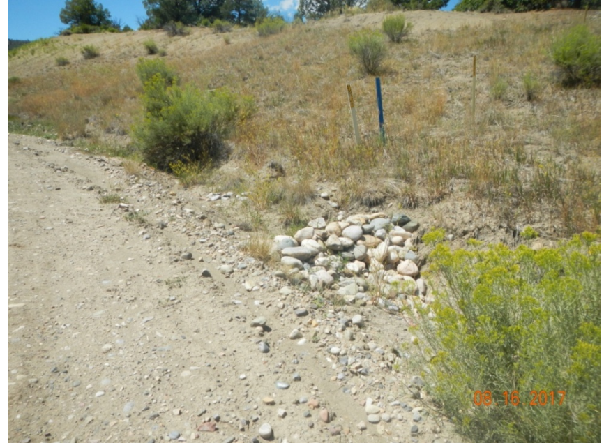
Photo 2: View of stormwater controls at the northern edge of the well pad entrance. Appear to be functioning.
