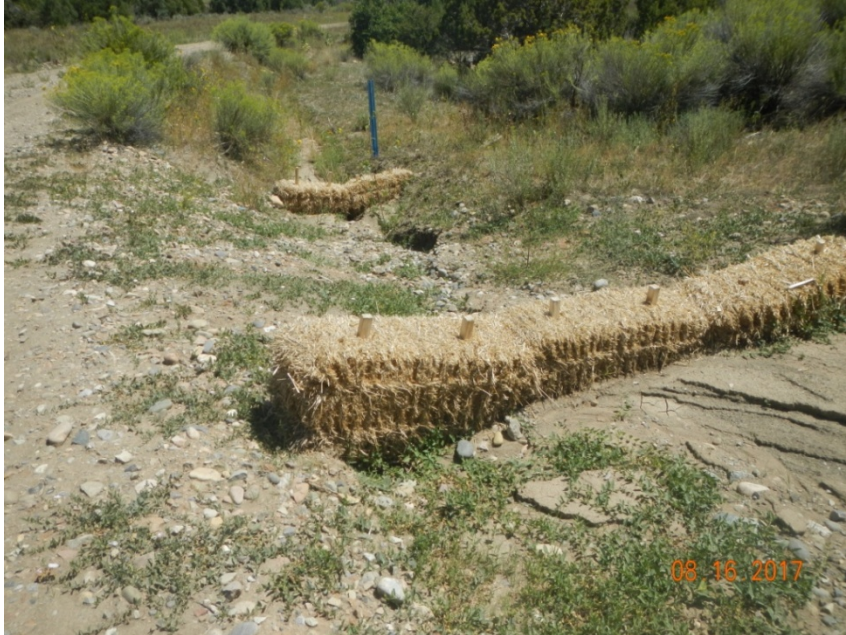
Photo 1: View of stormwater controls at the southern edge of the entrance to the well pad and access road. Need maintenance.
