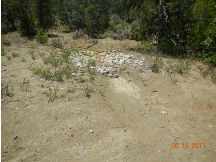
Photo 3: View of cobble run down along the northwestern edge of the project area appears to be functioning at this time.
