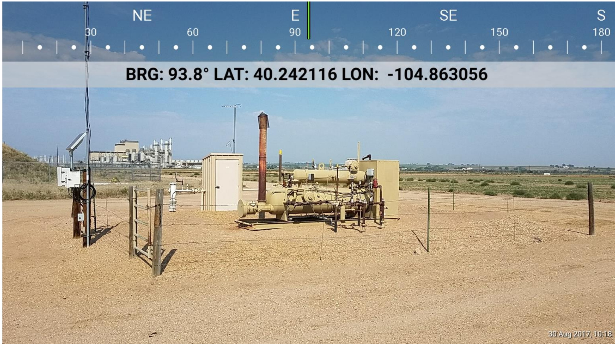
Separator and Gas Meter Run Location #: 329832
