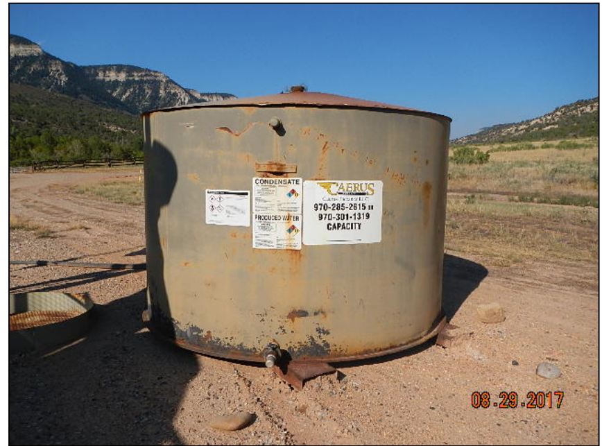
Photo 2. 100b Condensate Tank with no containment.
