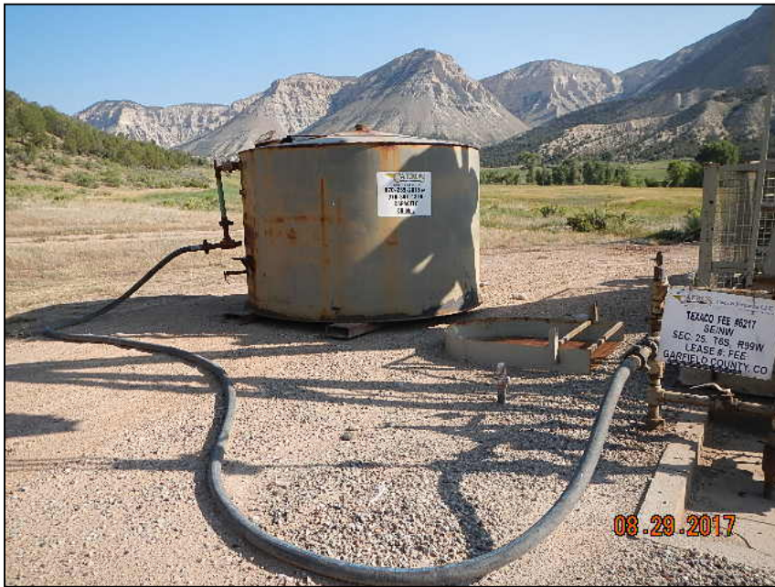
Photo 1. 100b Condensate Tank with no containment.
