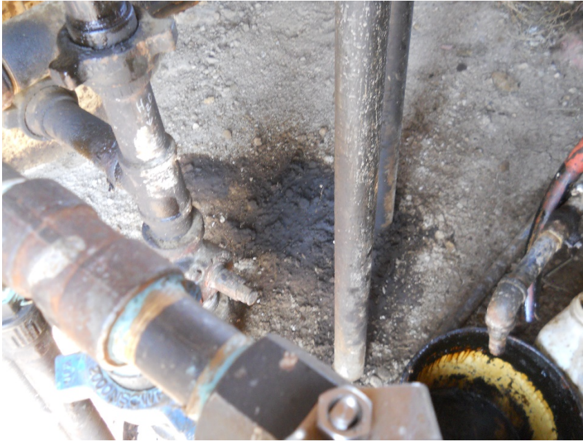
Stained soil in heater treater shed under oil leg from leaking valve
