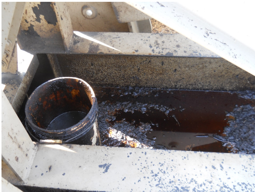
Stained soil in skid of pump jack, center. Standing fluid appears to be used motor oil. 5 gallon bucket approx. half full with what appears to be used motor oil. No wildlife protection
