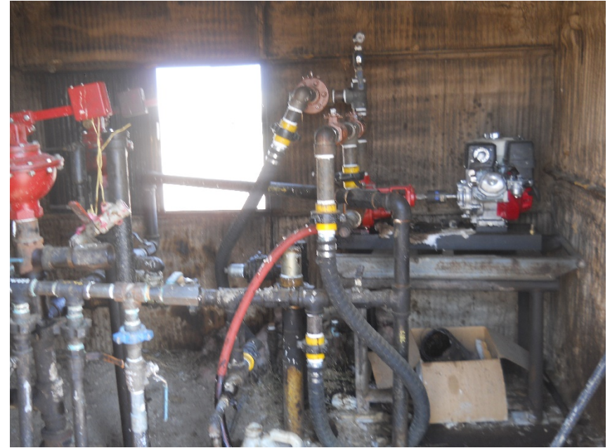
Circulating pump for tanks in heater treater shed
