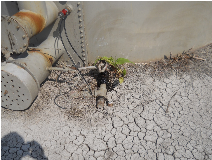
Leaking drain valve on south side of west crude oil tank
