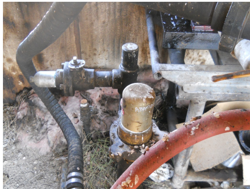
3" unused/marked steel riser, 2" unused/marked steel riser in heater treater. No LOTO
