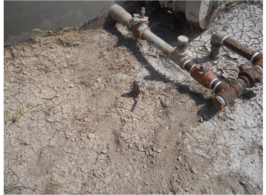
1-1" unused/unmarked steel riser south side of east middle produced water tank
