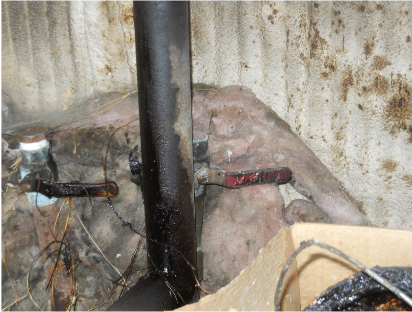
2-1" unused/unmarked steel risers north wall in heater treater shed
