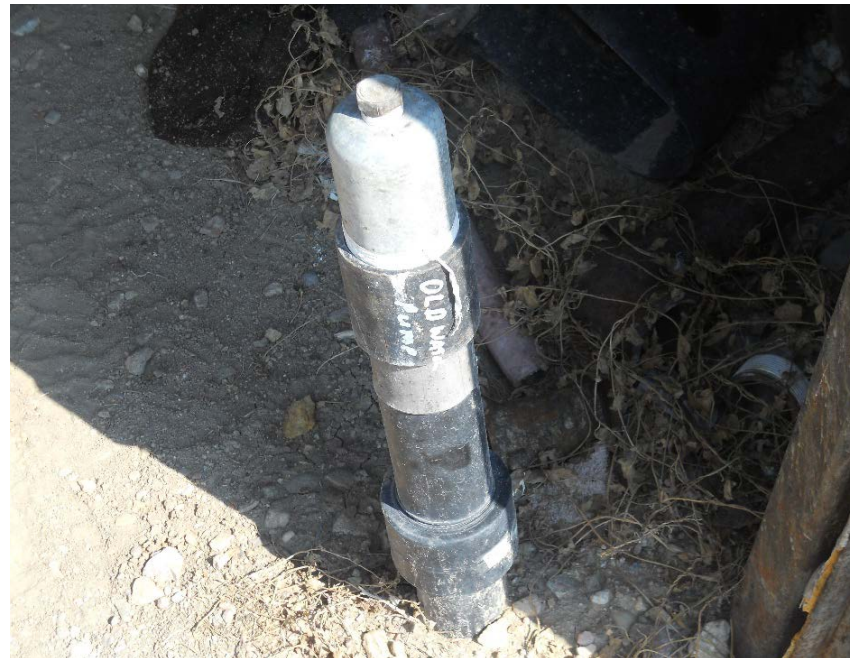
2" unused/marked poly line at heater treater shed entrance. No LOTO
