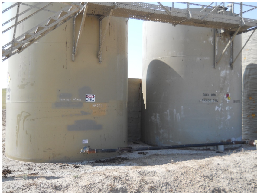
Produced water tanks looking south. East tank has correct labeling, west tank is labeled as crude oil and has produced water written under it. Uncertain of its contents. West tank needs NFPA label replaced.
