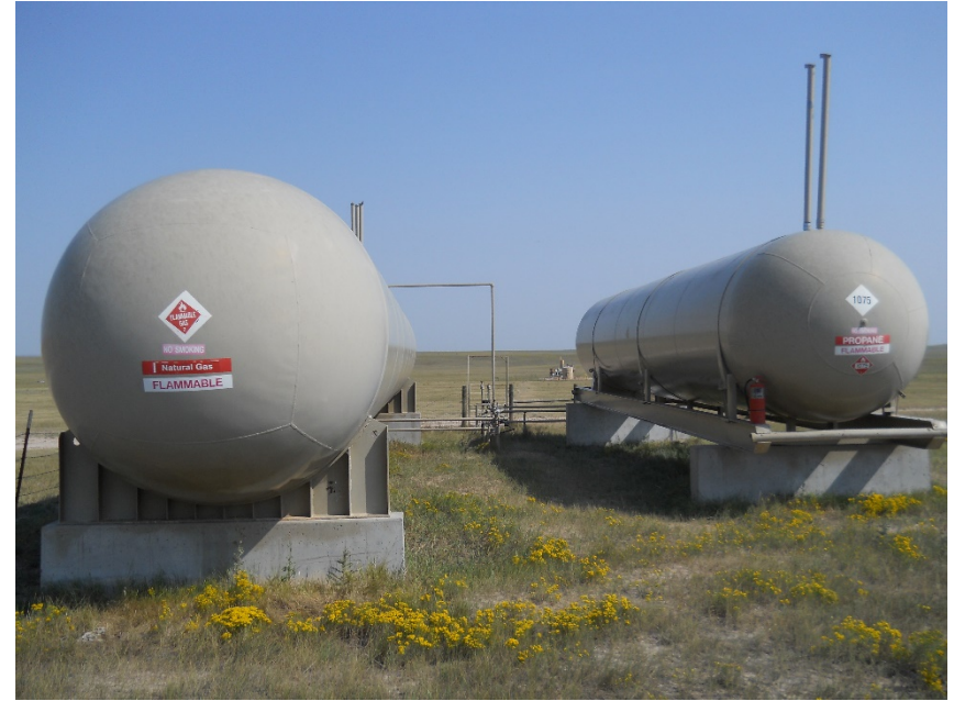
36,000 gallon natural gas tank and 18,000 gallon propane tank on northwest corner of location, looking north
