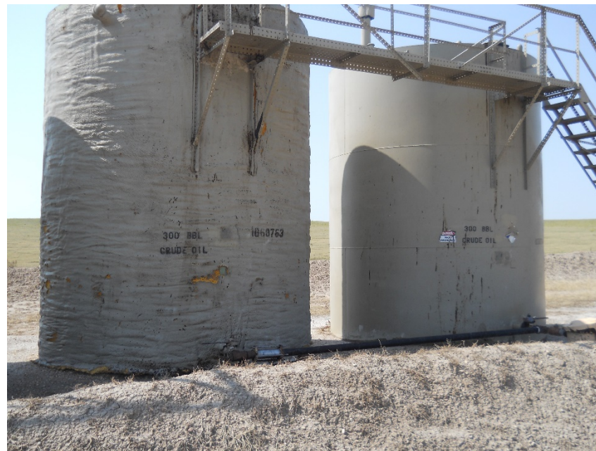
Crude oil tanks looking southwest. East tank has no NFPA label, west tank NFPA label not legible
