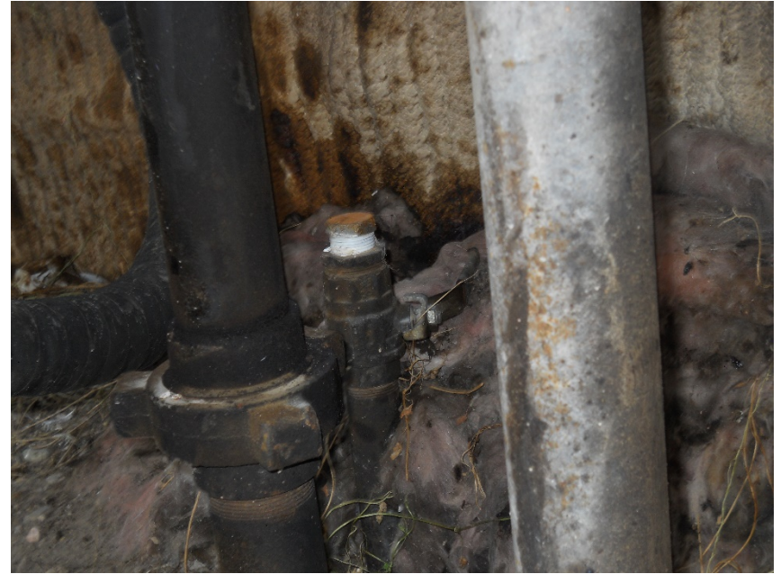
1-1" unused/unmarked steel riser north wall in heater treater shed
