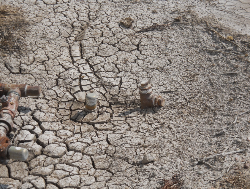
2-2" unmarked/unused steel risers south side of east produced water tank
