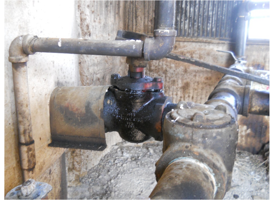
Leaking oil valve in heater treater
