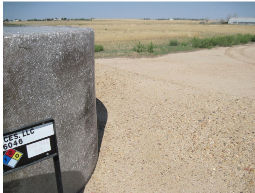
BERMS WILL NOT HOLD CAPACITY OF OIL PROD TANK
