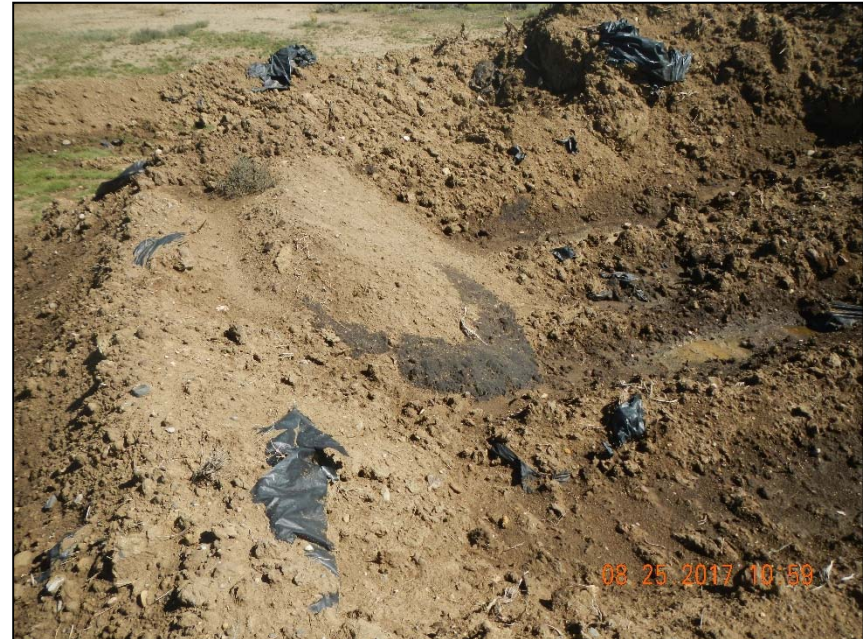
Photo 4. Close up. Land farm area with no containment. Berm around perimeter is unconsolidated and contains pieces of debris.
