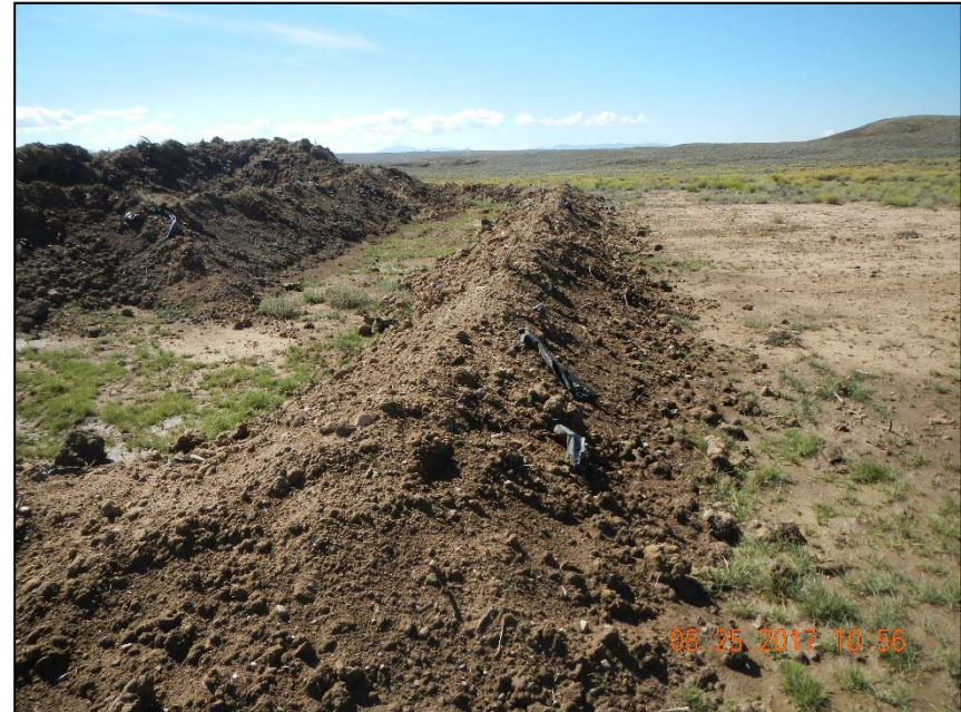
Photo 2. Land farm area with no containment. Berm around perimeter is unconsolidated and contains pieces of debris.
