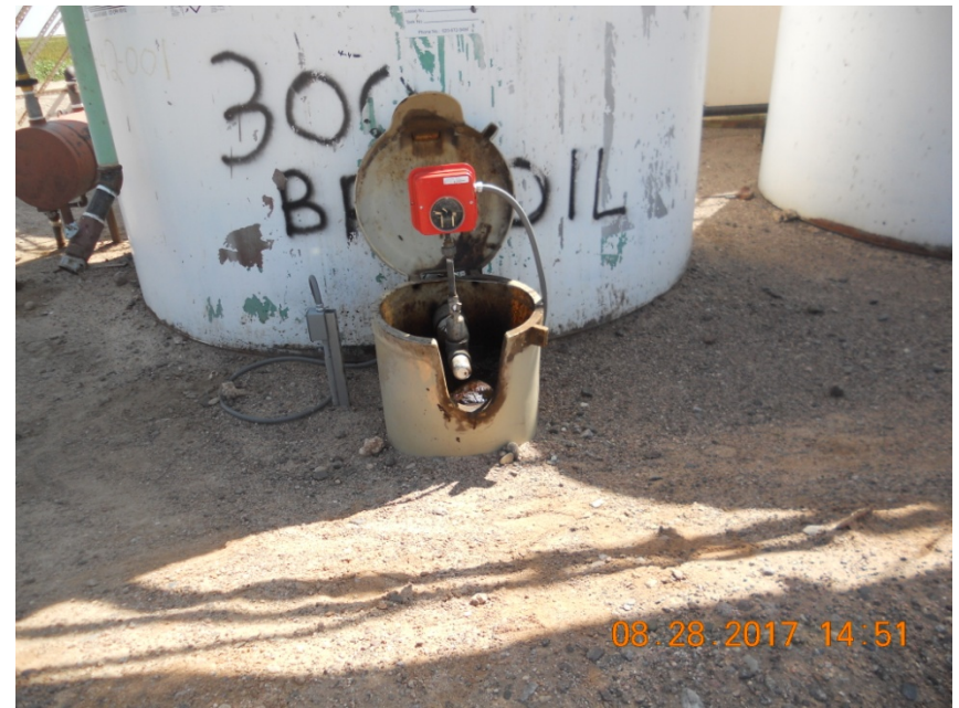
Photo 2. Containment device full of liquid and open
