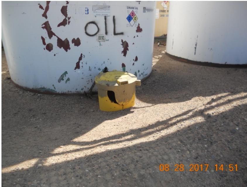
Photo 1. Containment equipment broken can allow wildlife intrusion
