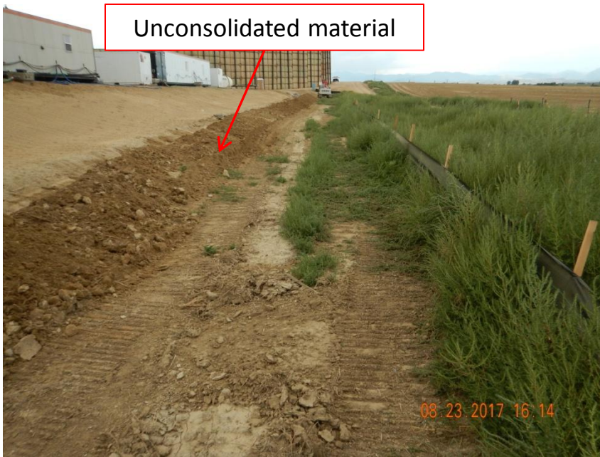
Photo 13. Photo taken from the northwestern location, facing West. Ditch installed along the pad perimeter with check dams, but unconsolidated material needs to be stabilized. Silt fence installed around the western and a portion of the southern location. Fill slopes have been tracked perpendicular with equipment for temporary stabilization.
