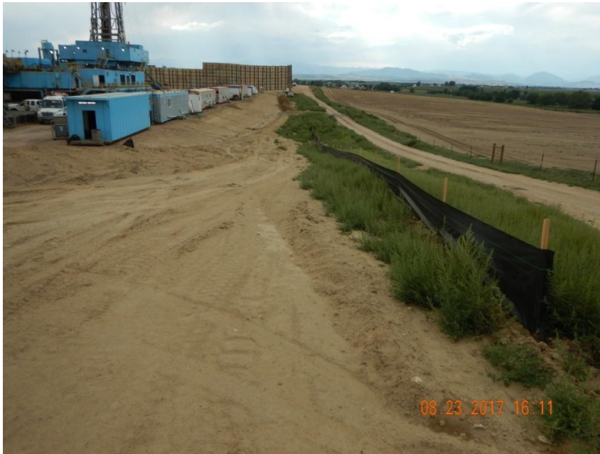
Photo 11. Photo taken from the northeastern location, facing West. Ditch installed along the pad perimeter with check dams. Silt fence installed around the western and a portion of the southern location. Fill slopes have been tracked perpendicular with equipment for temporary stabilization.
