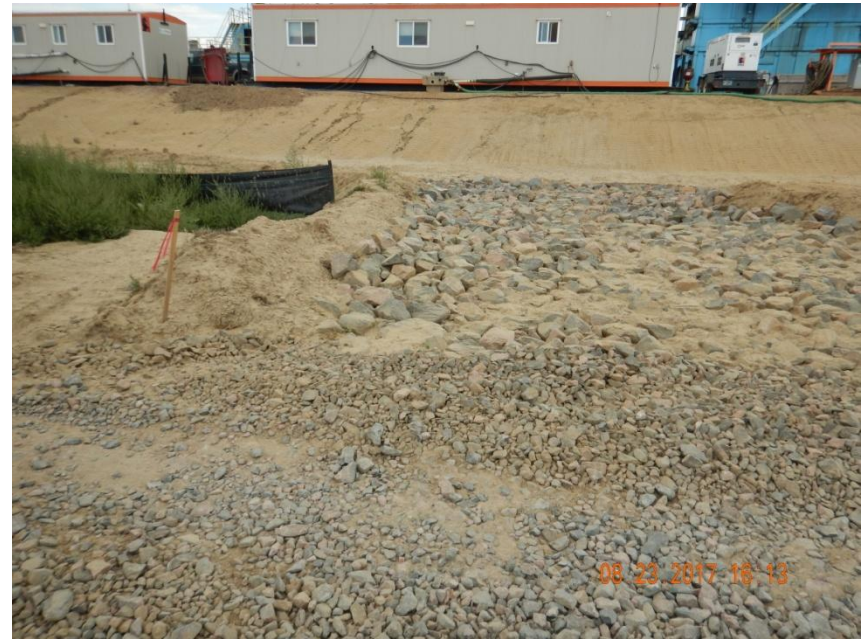
Photo 12. Photo taken from the north-central location, facing South. A stabilized area constructed of rip-rap has been installed for erosion control. However, this may not be considered a sufficient sediment control BMP, especially as sediment builds up within the rip-rap. More rip-rap was observed on the other side of the access road but, again, that may not be sufficient as a sediment control BMP.
