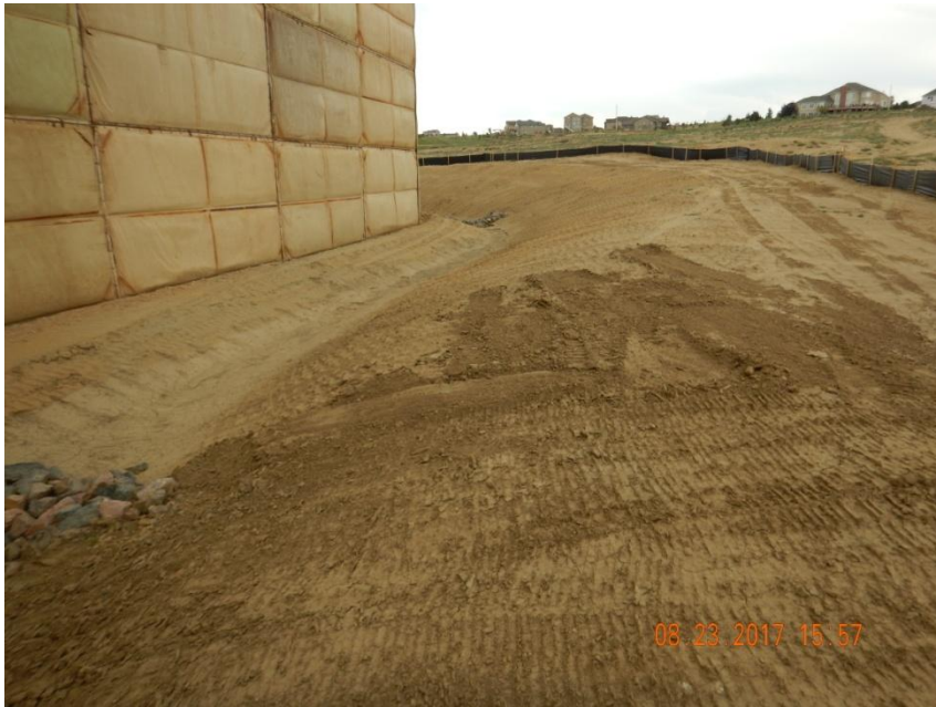
Photo 5. Photo taken from the western location, facing South. Ditch installed along the pad perimeter with check dams. Silt fence installed around the western and a portion of the southern location. Cut slopes have been tracked perpendicular with equipment for temporary stabilization.
