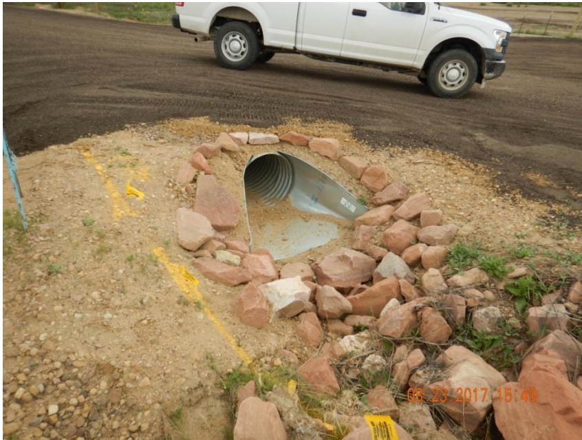
Photo 3. Photo taken from the entrance of location, facing North. Culvert installed along burrow ditch with stabilized inlet and outlet devices.
