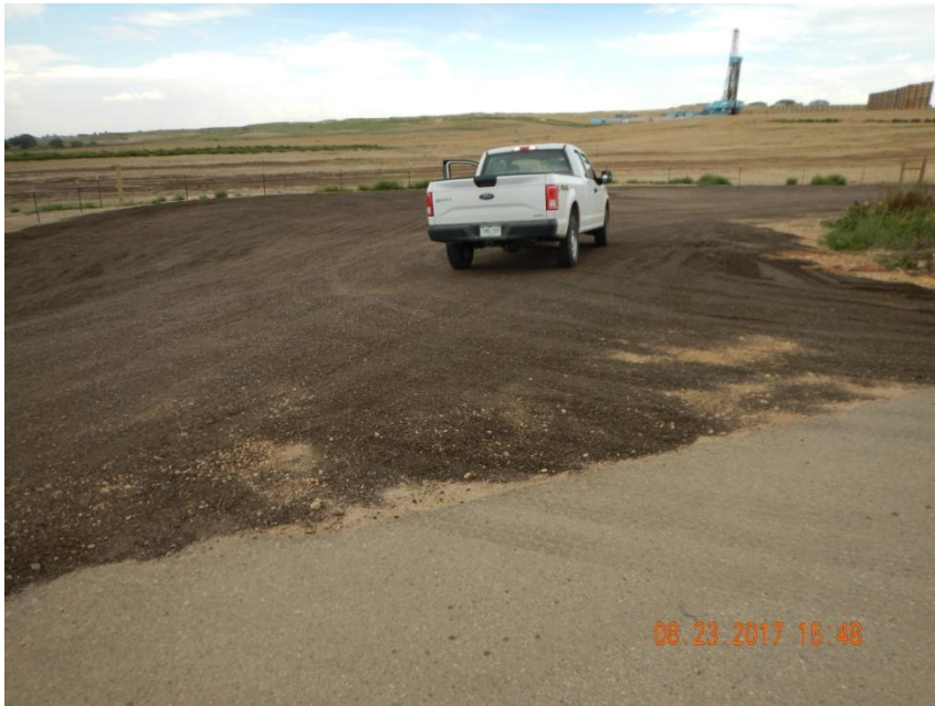
Photo 1. Photo taken from the entrance of location, facing East. Tracking pad devices installed at location- see next photo for more tracking pad BMPs.
