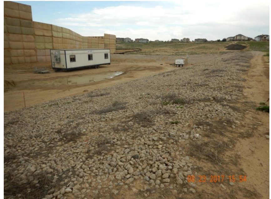
Photo 4. Photo taken from the northwest location, facing South. Cut slopes have been stabilized with rock material.
