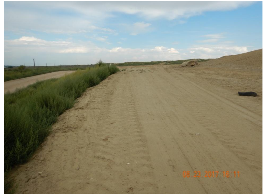
Photo 10. Photo taken from the northeastern location, facing East. There were no erosion and/or sediment control BMPs along this area. This area has potential for stormwater runoff.
