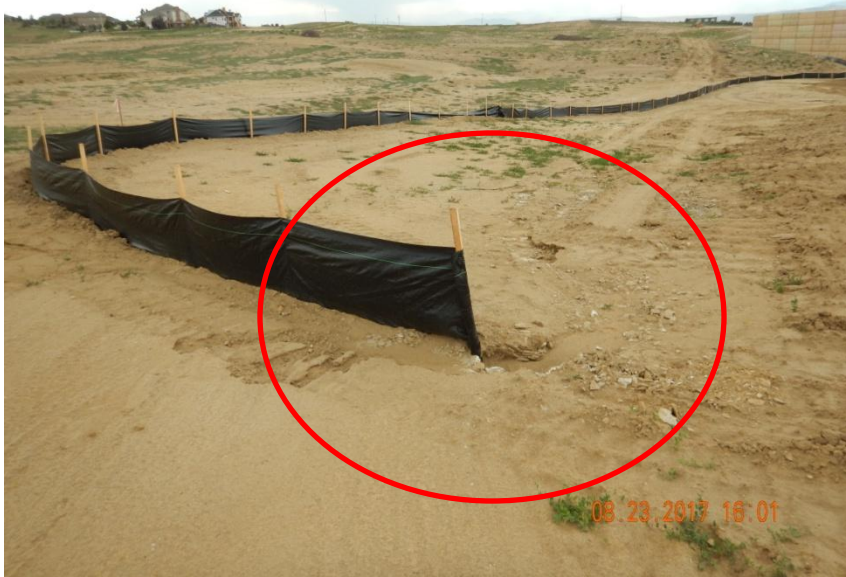
Photo 7. Photo taken from the southern location, facing West. A point of run-on onto location was observed right at the stopping point of the silt fence.
