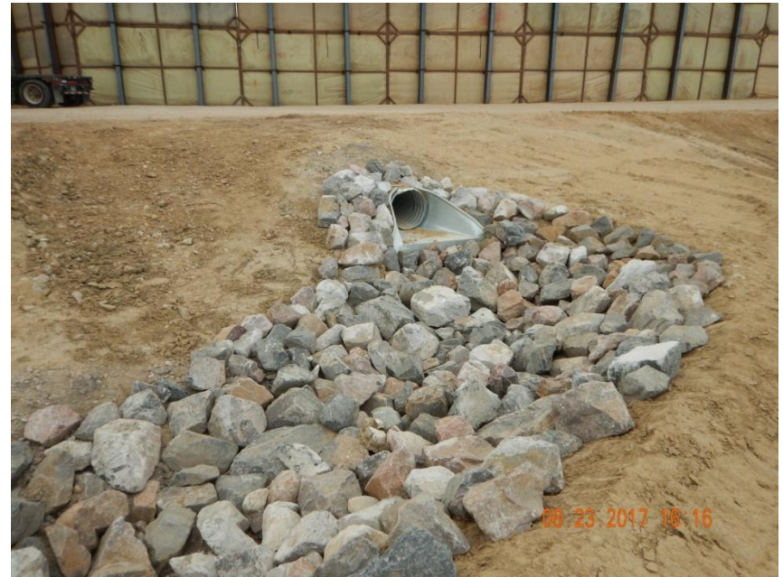
Photo 14. Photo taken from the northwest location, facing South. A stabilized outlet from a culvert installed in conjunction with the ditch BMP.
