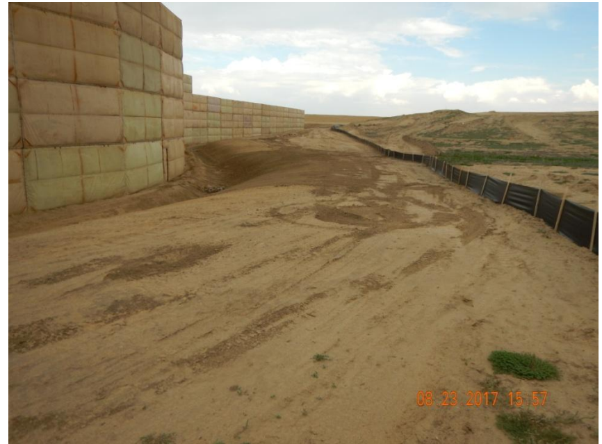
Photo 6. Photo taken from the southwestern location, facing East. Ditch installed along the pad perimeter with check dams. Silt fence BMP installed around the western and southern location. Cut slopes have been tracked perpendicular with equipment for temporary stabilization.
