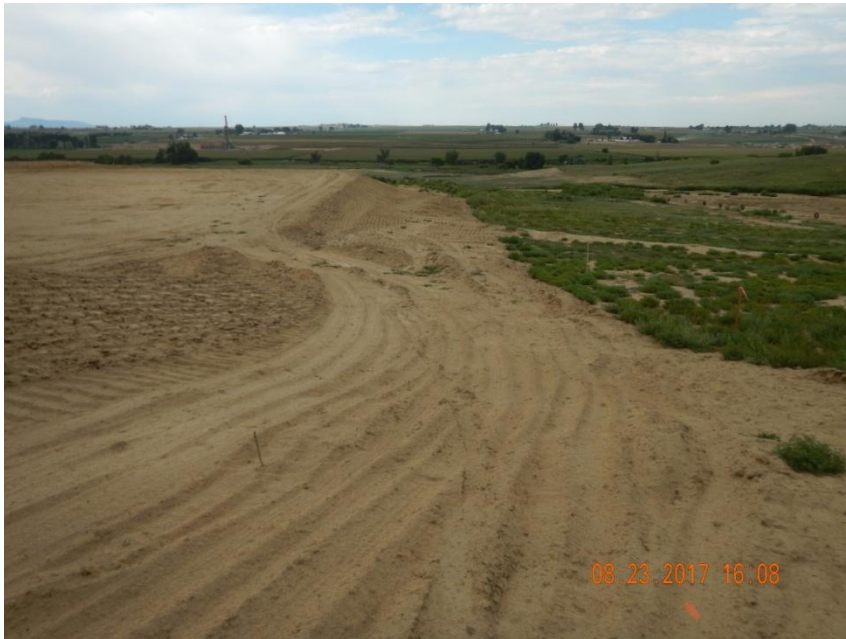
Photo 9. Photo taken from the southeastern location, facing North. There were no erosion and/or sediment control BMPs along the eastern location. The eastern location has potential for stormwater runoff, as minor rill erosion was observed.
