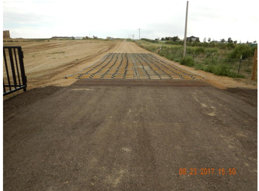
Photo 2. Photo taken from the entrance of location, facing South. Tracking pad devices installed at location.
