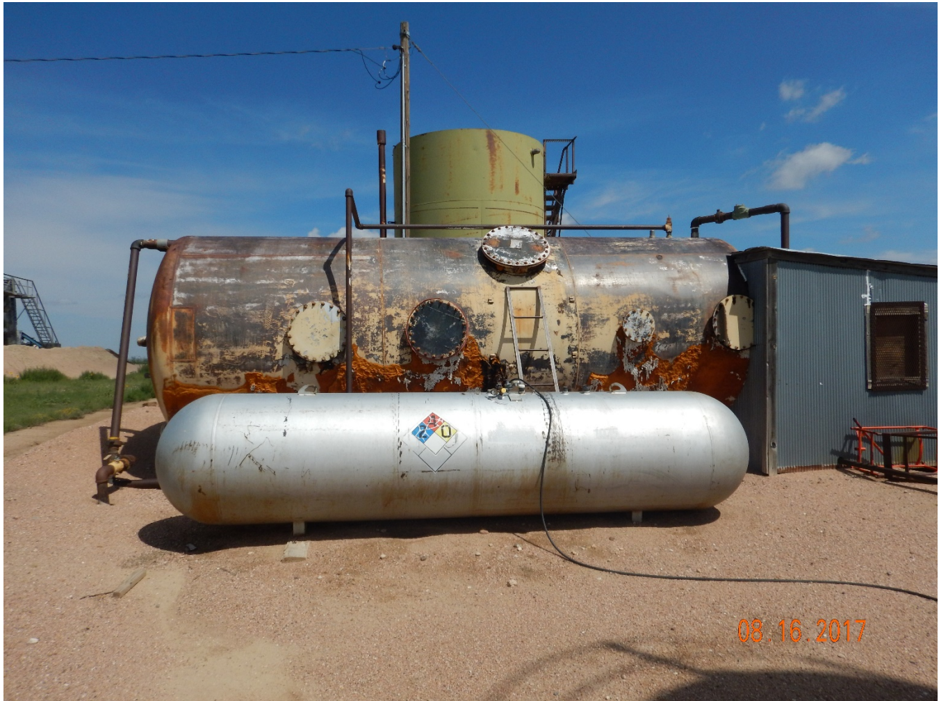
Figure 9 - Unlabeled horizontal AST/FWKO and propane tank south of produced water AST.
