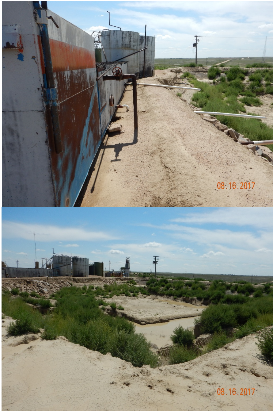
Figure 18 - Produced water tanks share earthen berm (and are plumbed to) active pit facility #107647.
