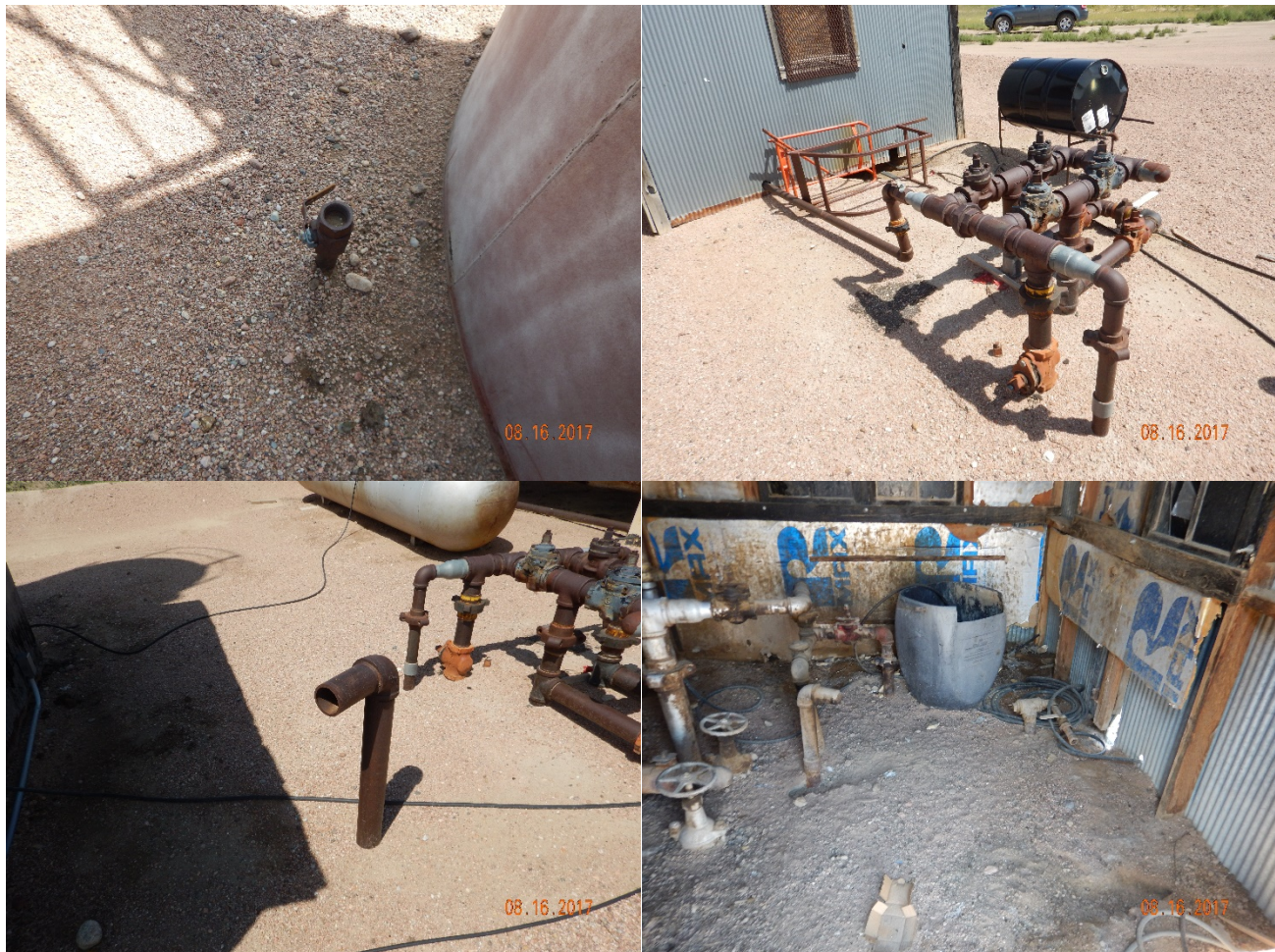
Figure 12 - Flowline risers around crude oil tank battery. Clockwise from top left: 2" uncapped line north of crude oil tanks, manifold and storage drum south of FWKO, two 2" risers inside of VHT shed and 4" riser with 90-degree angle south of manifold.
