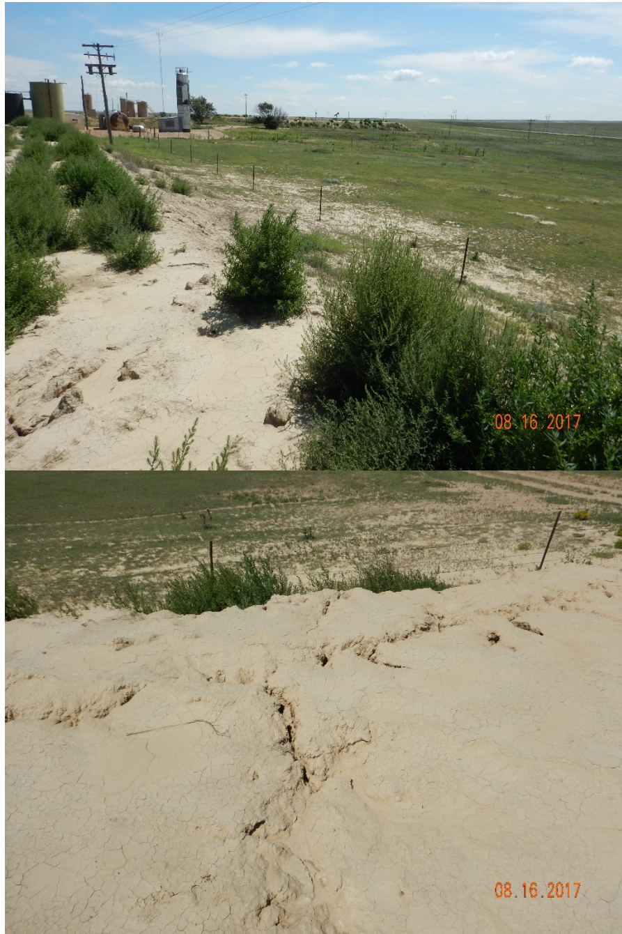
Figure 19 - Evidence of berm erosion and off-site sediment transport to south (top photo) and west (bottom photo) of pit facility #107647.
