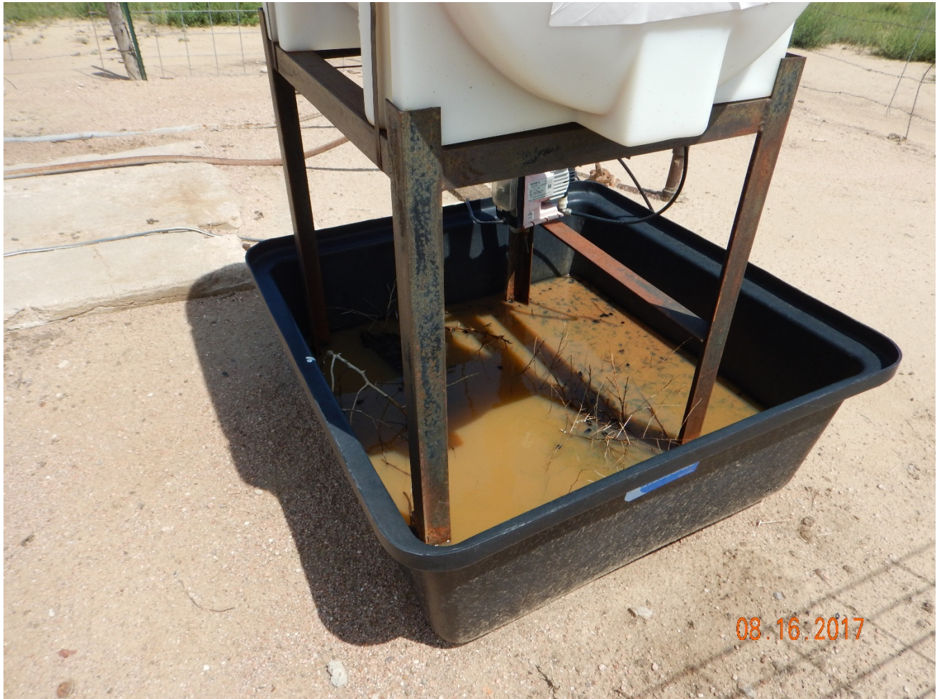
Figure 3 - Day tank with secondary containment device at wellhead. Note presence of contaminated stormwater inside of containment device.
