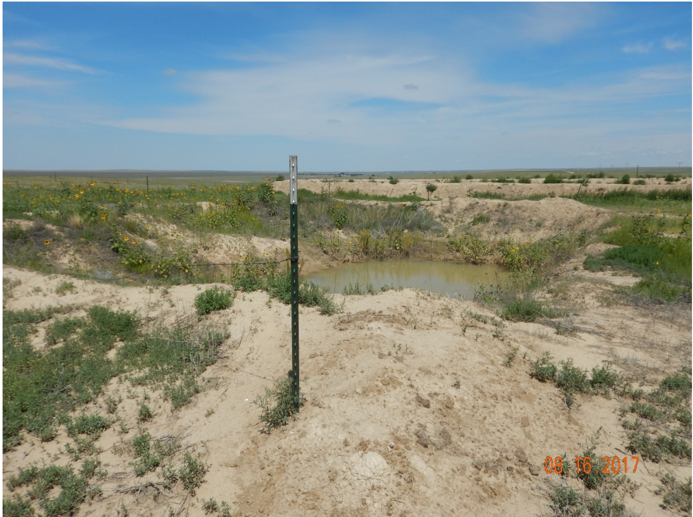
Figure 21 - Open excavation associated with skim pit closure (facility IDs #107645 & #107646) and Remediation Project #8068 remains open, is overgrown with weeds, and is partially filled with water. Fence in need of repair.
