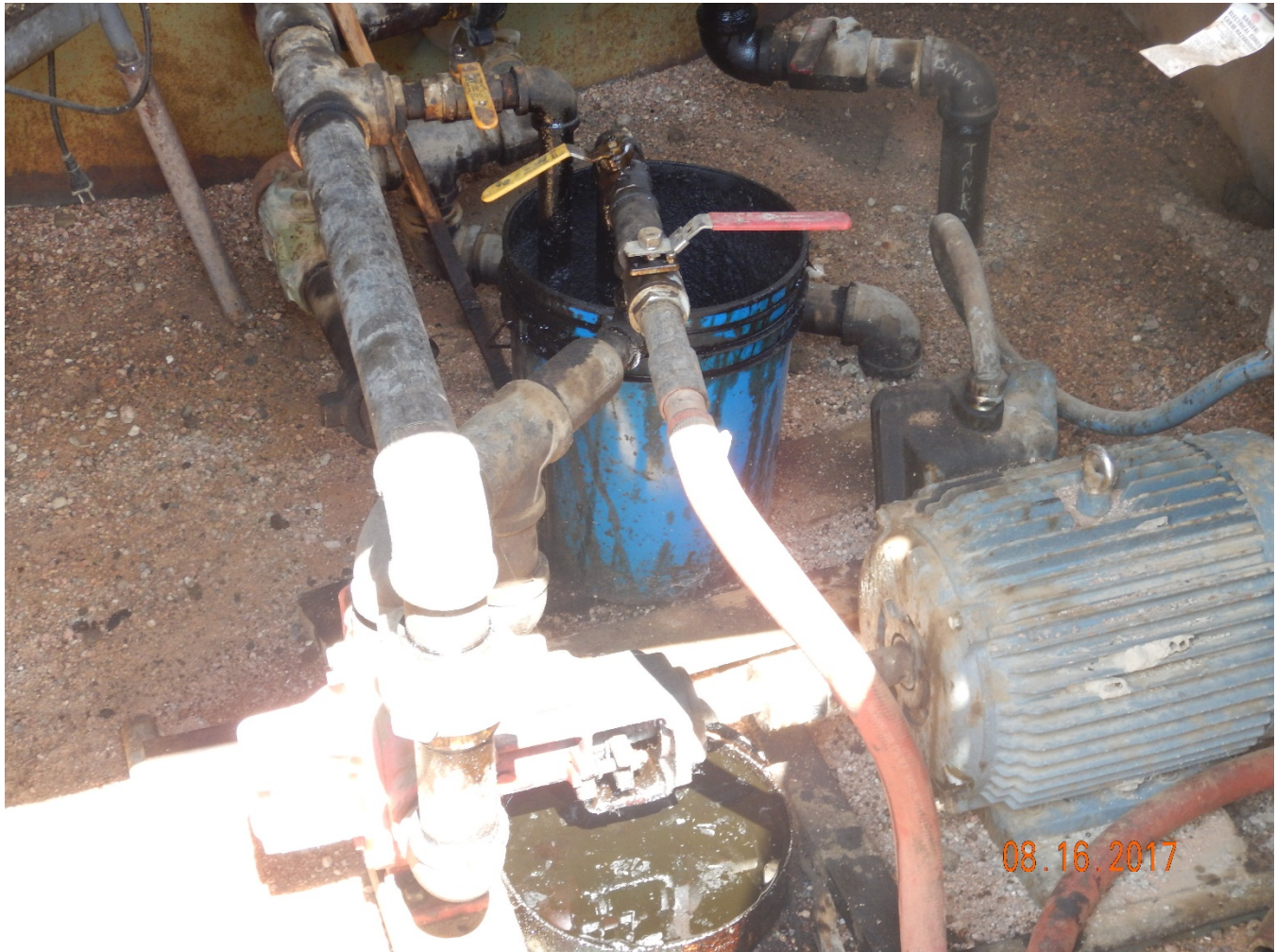
Figure 8 - Open buckets of oily waste and oil-stained soil inside of shed attached to 400 bbl produced water AST.
