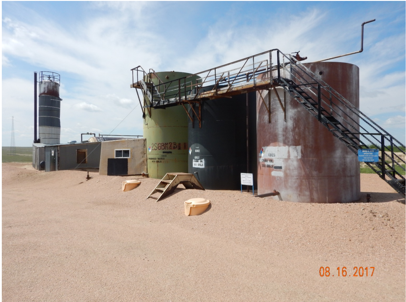
Figure 5 - Crude oil battery with FWKO and VHT.
