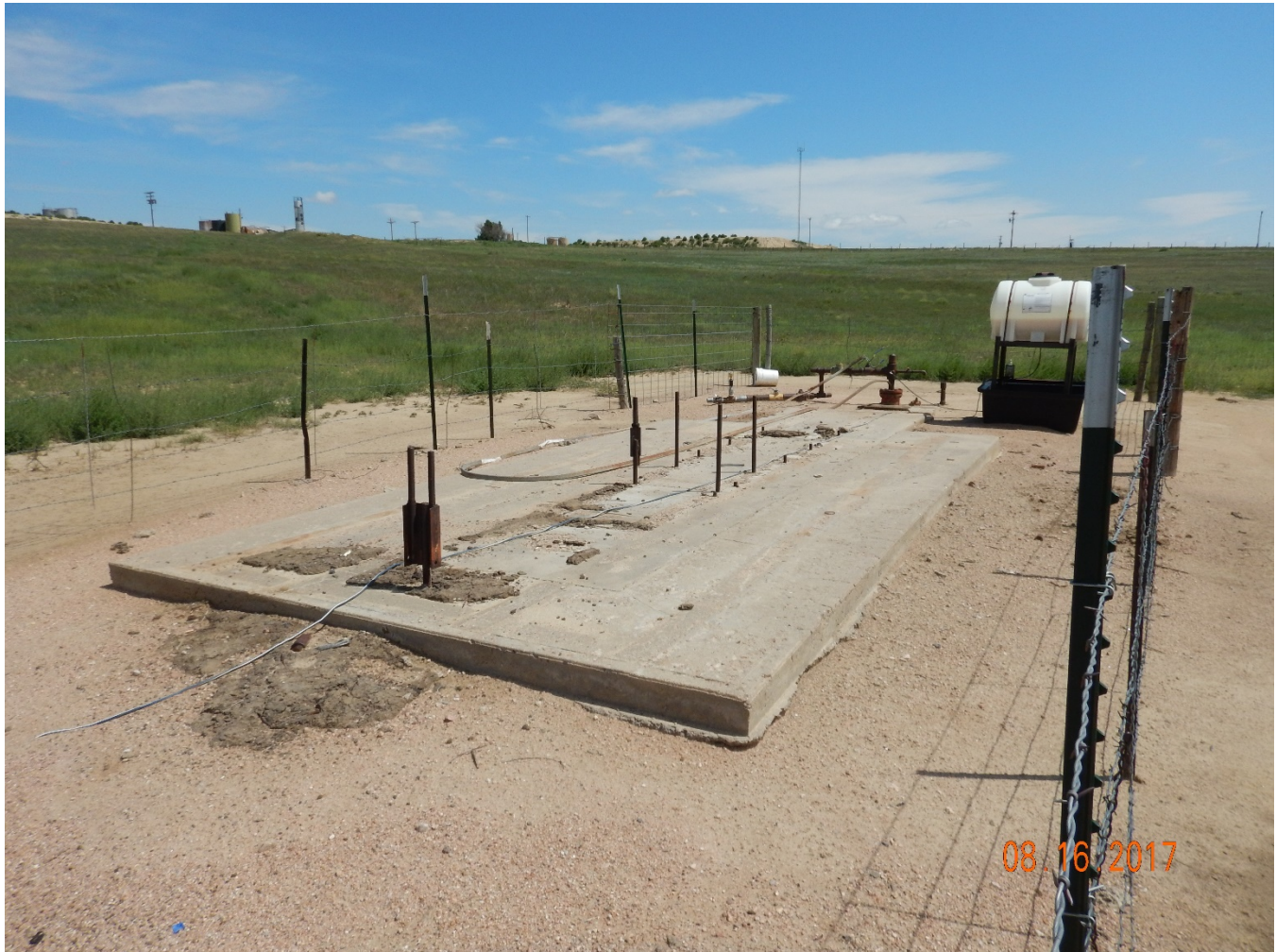
Figure 2 - Pump jack foundation and wellhead. Note presence of oily waste associated with pump jack foundation.
