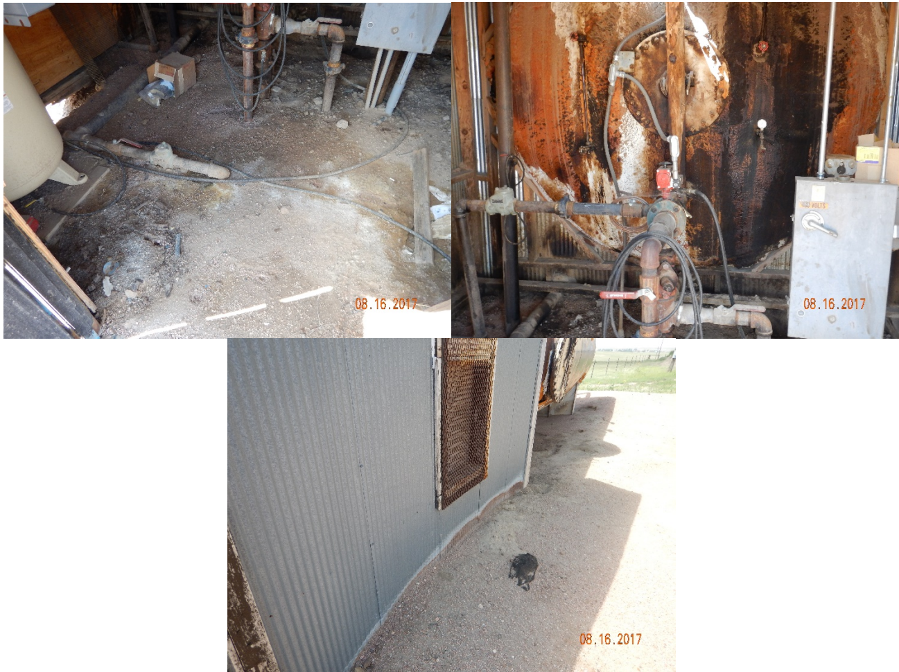
Figure 10 - Oil-stained soil and equipment (top photos) inside of FWKO shed and oily rag outside of window on north side of shed (bottom photo).
