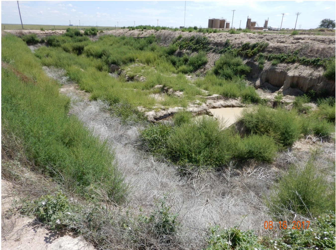
Figure 24 - View of active pit facility #117577 from NW corner. Note abundance of weeds and oil-stained soil above water line in foreground.
