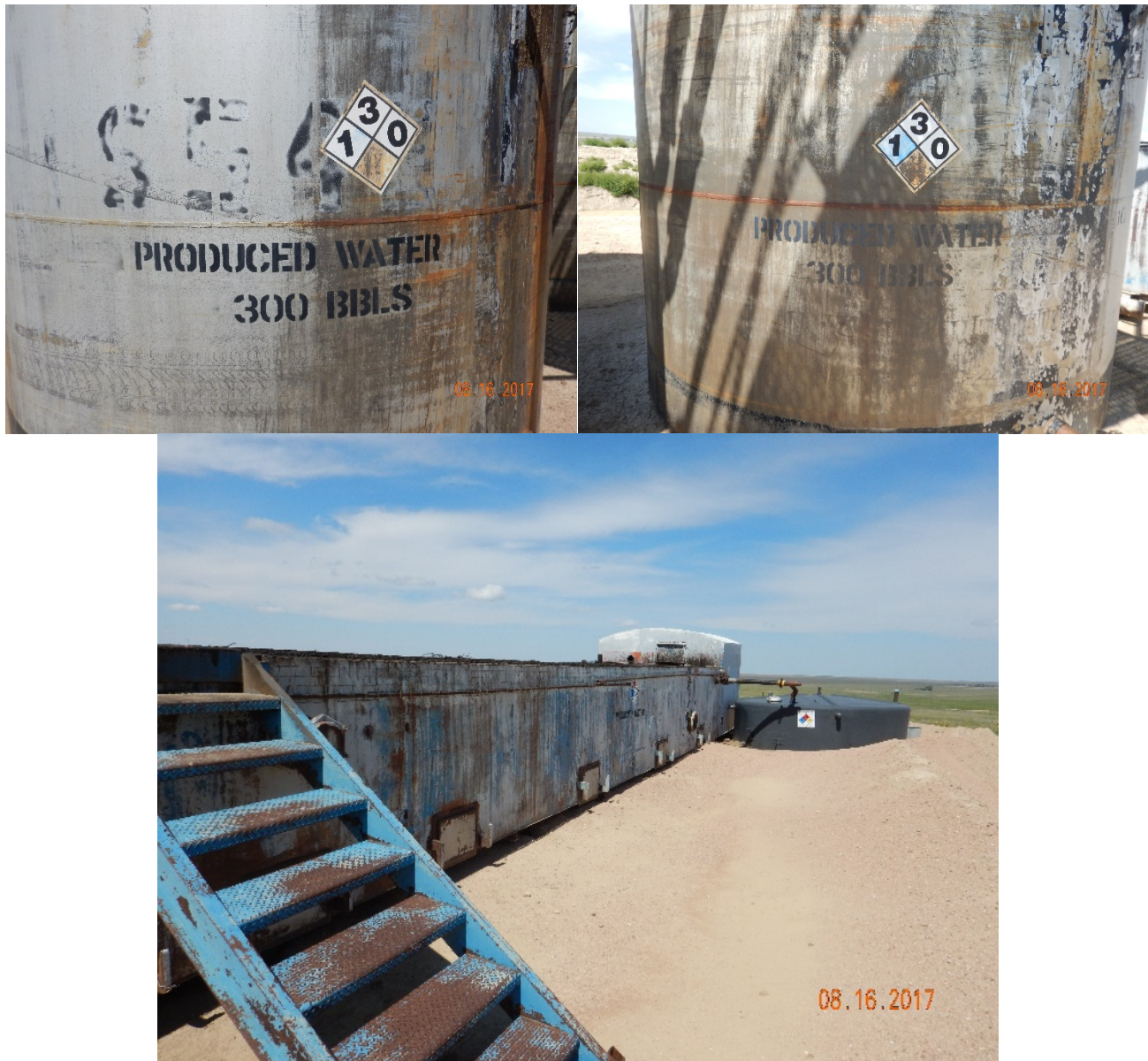
Figure 17 - Placard and label issues with produced water tanks: Top photos: 300 bbl ASTs have faded NFPA placards and labels are illegible from a distance due to tank color and stains. Bottom photo: frac tank and PBV have NFPA placards but no volume labels.
