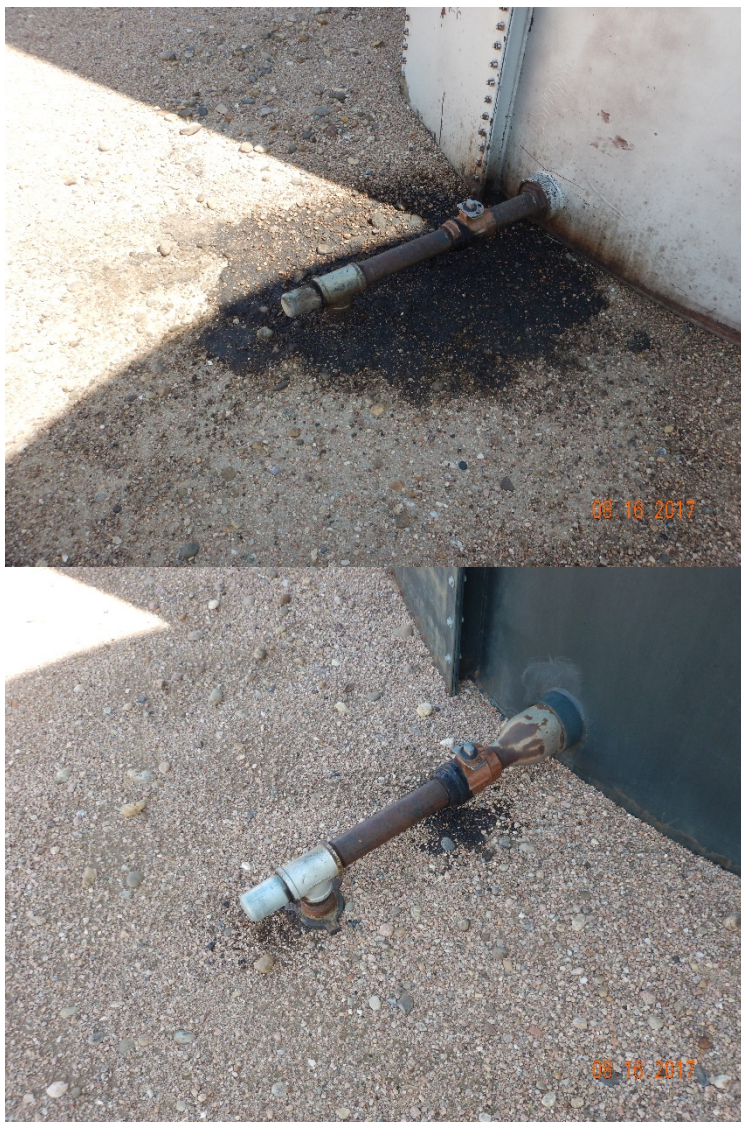
Figure 6 - Oily waste underlying valves on west side of crude oil ASTs.
