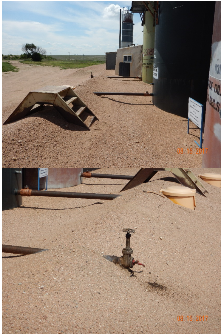
Figure 7 - Shallow earthen berm (top photo) and oily waste at truck loadout (bottom photo).
