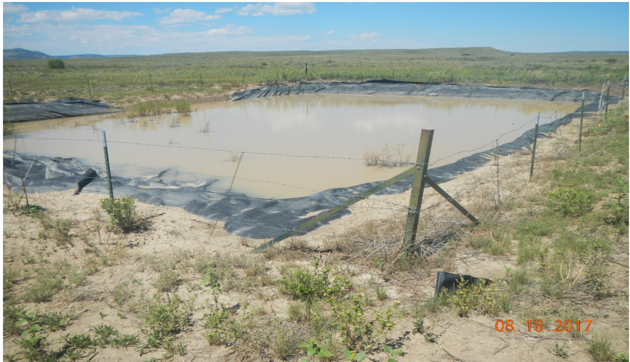
photo 3: The northeast toward the pit. The liner appears to be degraded and the fence around the pit is not maintained.
