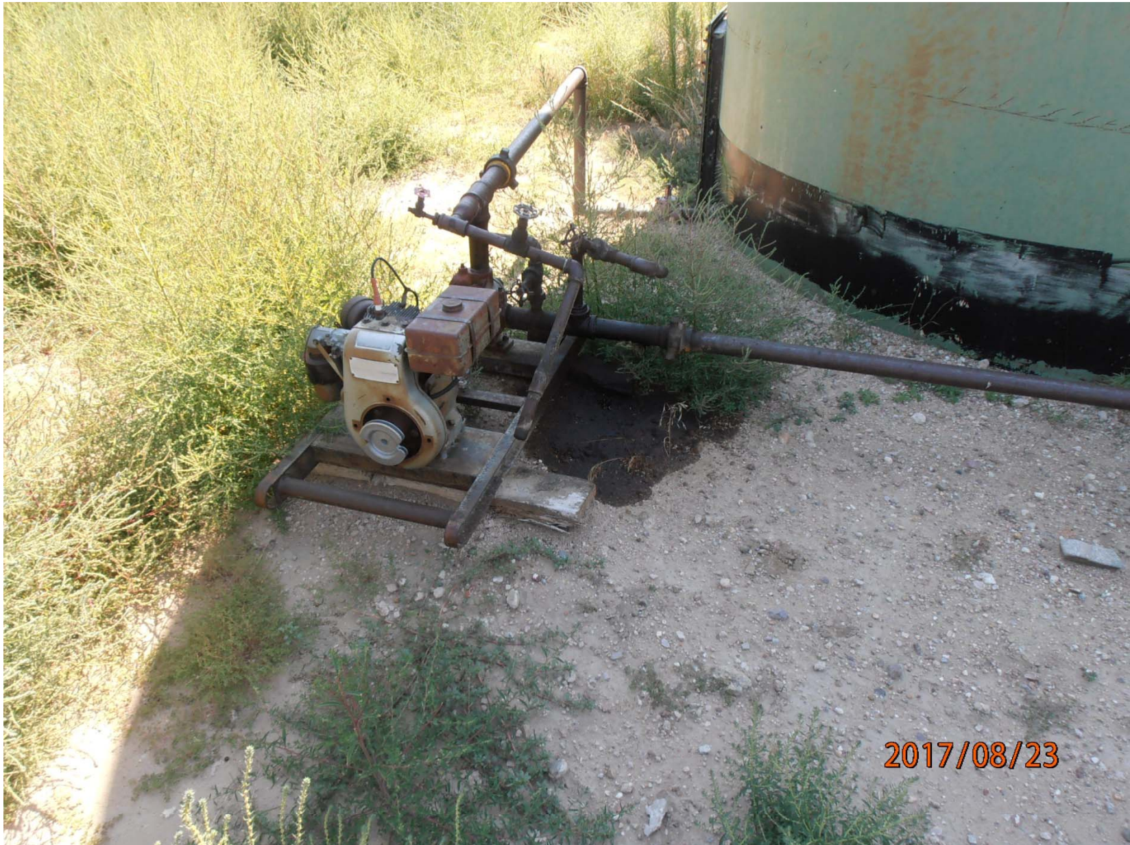
Crude oil leak at transfer pump
