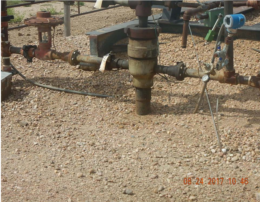
Photo 3: Bradenhead not plumbed to surface
