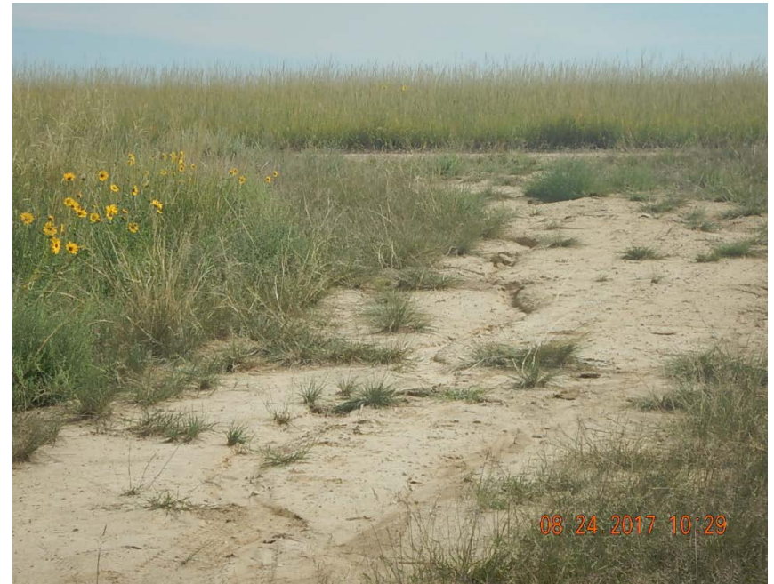
Photo 2: Stormwater erosion on lease road, looking E
