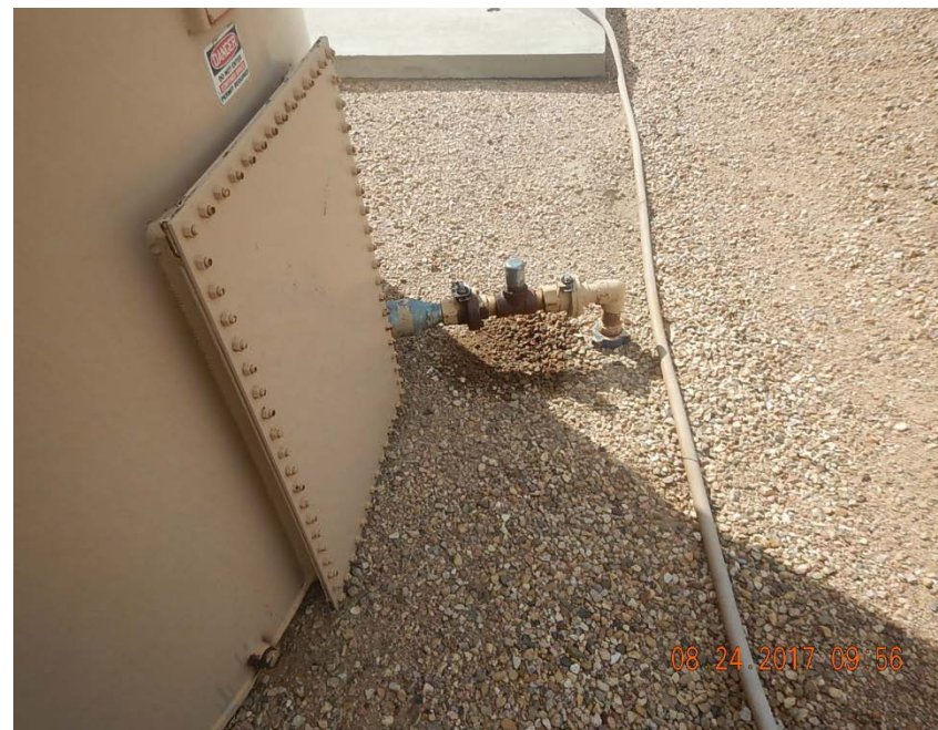
Photo 4: Stained soil at valve
