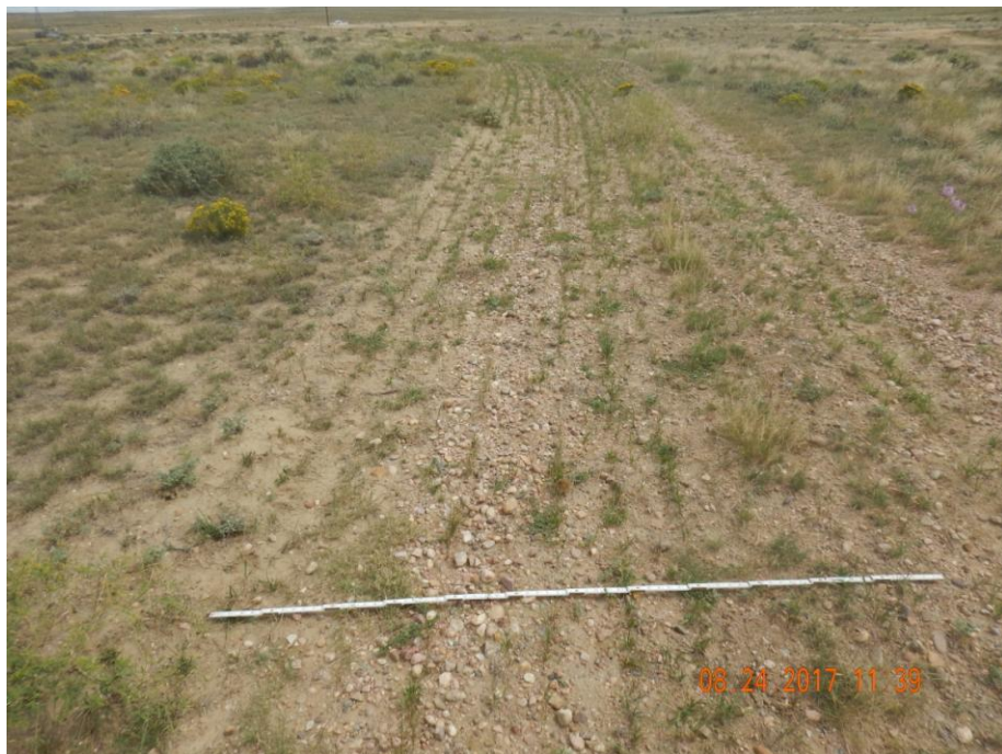
Photo 5: Photo taken from the from the access road, north of the location facing north. Previous inspection required operator to remove gravel/road base from the access road, perform compaction alleviation, re-contour/re-grade. Photo shows gravel/road base remains on access road. No additional reclamation activities per CA's have been conducted. 6 foot measuring stick for reference.
