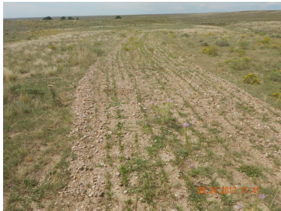
Photo 6: Photo taken from the from the access road, north of the location facing south. Previous inspection required operator to remove gravel/road base from the access road, perform compaction alleviation, re-contour/re-grade. Photo shows gravel/road base remains on access road. No additional reclamation activities per CA's have been conducted.
