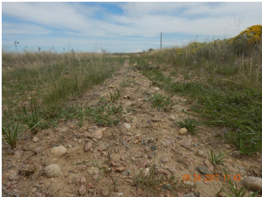
Photo 9: Photo taken from the access road, facing north. Photo shows gravel/road base remaining on location. Photo also shows access road had not been re-contoured or re-graded on large sections of the road to match the adjacent reference area.
