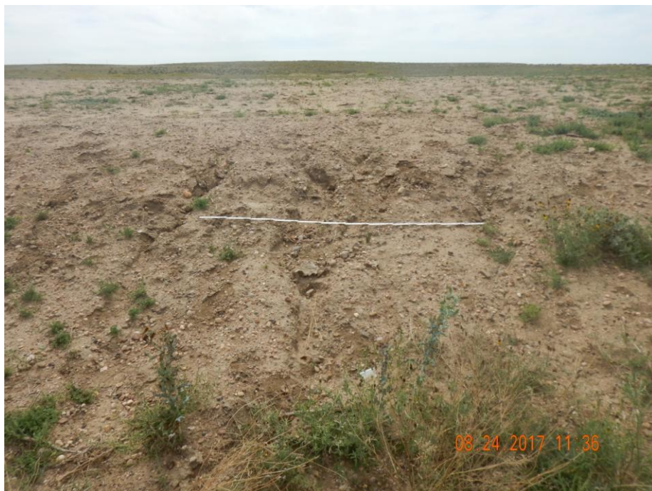
Photo 3: Photo taken from the west end of the location. Photo shows stormwater erosion. Previous inspections required operator to repair erosion and install controls to mitigate future stormwater erosion and degradation from occurring. Erosion was once repaired in this area, however no stormwater BMPs were installed or maintained and degradation has been allowed to persist. 6 foot measuring stick for reference.
