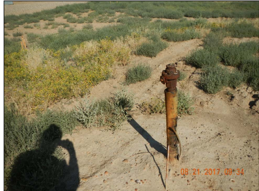
Photo 4. Not marked not LO/TO steel riser at 40.70062, -107.55674
