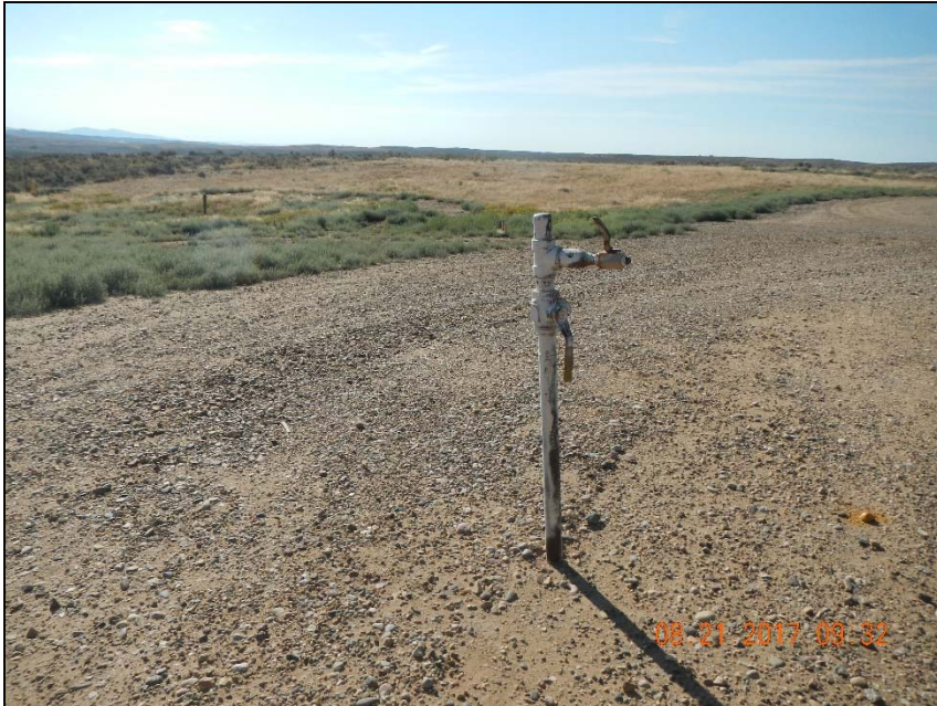
Photo 3. Not marked not LO/TO steel riser at 40.70078, -107.55706
