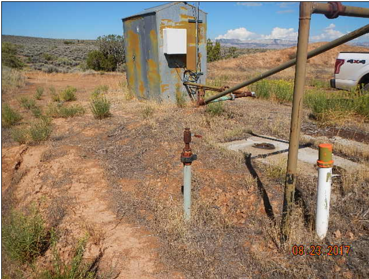
Photo 1. Unmarked 2" riser @ 39.226819/-108.238964
