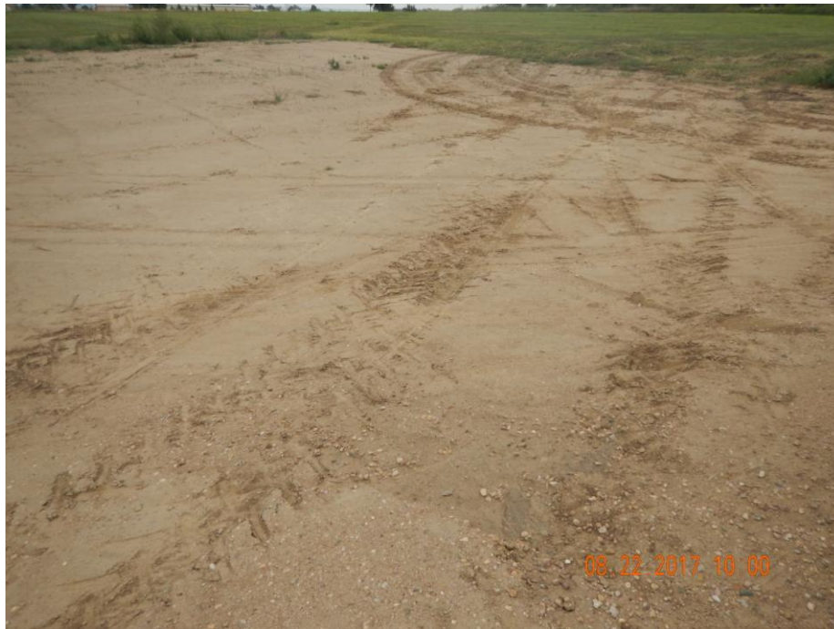
Photo 1: Photo taken from the center of the location, facing northeast. Photo shows the gully formations on the north half of the location have been repaired. However, no BMPs have been installed to mitigate future stormwater degradation concerns.
