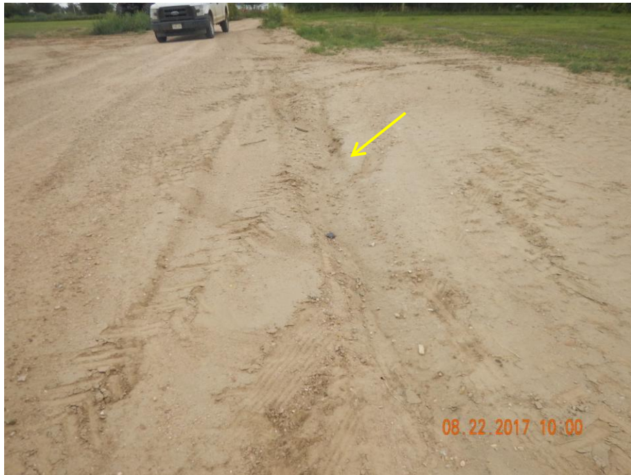
Photo 3: Photo taken from the south central area of the location, facing east. Photo shows the gully formations are beginning to form again on the southern end of the location. No BMPs have been installed to mitigate stormwater degradation concerns
