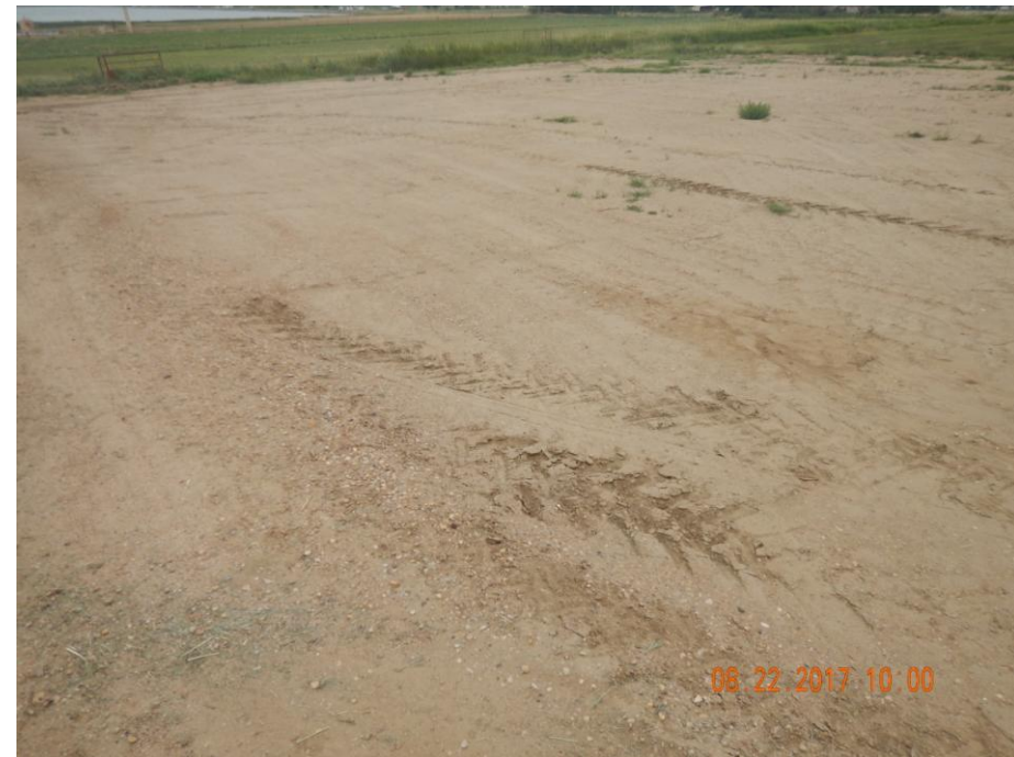
Photo 2: Photo taken from the center of the location, facing southwest. Photo shows the gully formations on the north half of the location have been repaired. However, no BMPs have been installed to mitigate future stormwater degradation concerns.
