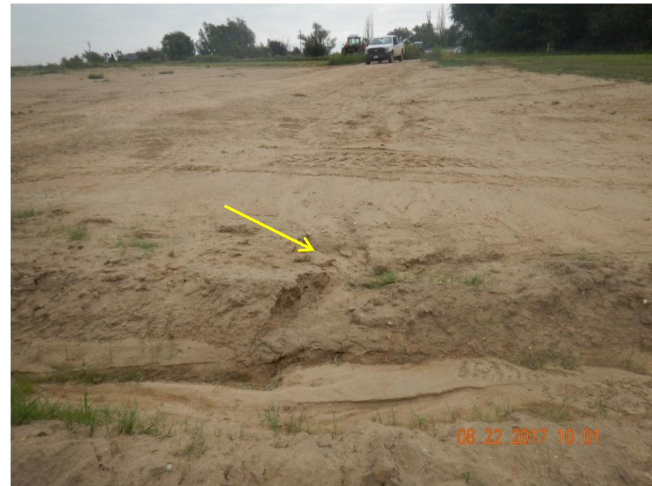
Photo 4: Photo taken from the ditch that runs North/South on the west end of the location, facing east. It is unclear if ditch had been repaired since previous inspection; stormwater degradation remains evident and sediment laden storm water discharge from the location is being deposited into the irrigation ditch.
