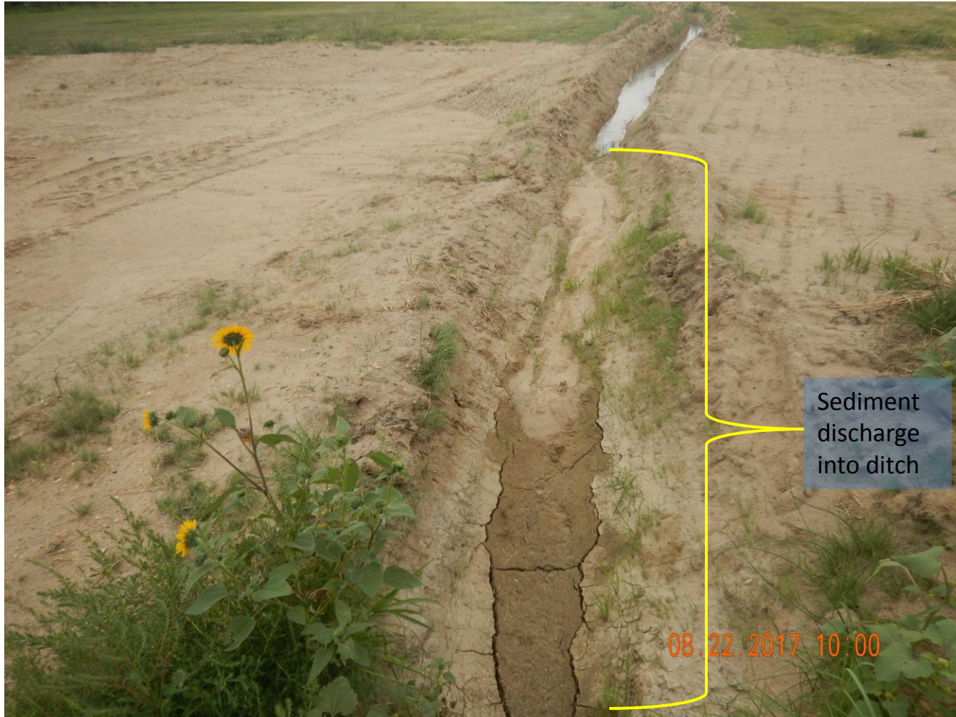
Photo 5: Photo taken from the ditch that runs North/South on the west end of the location, facing north. It is unclear if ditch had been repaired since previous inspection; stormwater degradation is remains evident and sediment laden storm water discharge from the location is being deposited into the irrigation ditch.
