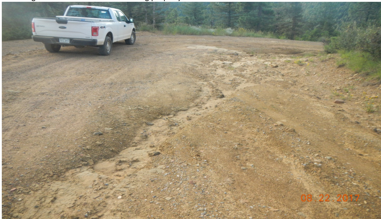
photo 2: Facing down the road Stormwater is flowing down the road causing erosion.
