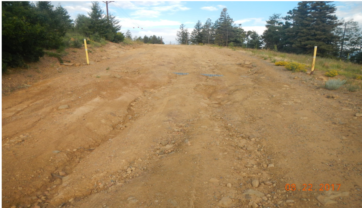
photo 1: Facing west along the main road. There is signs of erosion along the road. Stormwater water is flowing down the road and is not being properly diverted.
