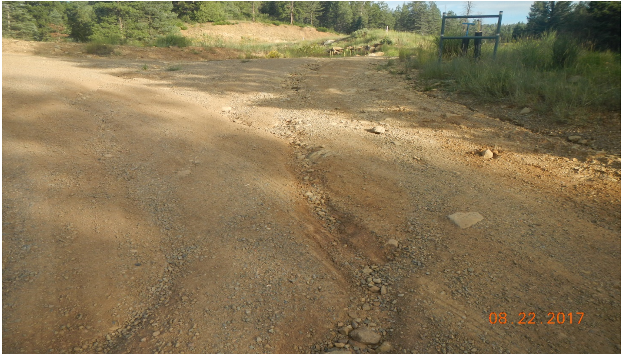
photo 1: Facing west along the main road. There is signs of erosion along the road. Stormwater water is flowing down the road and is not being properly diverted. Road base material has eroded away.
