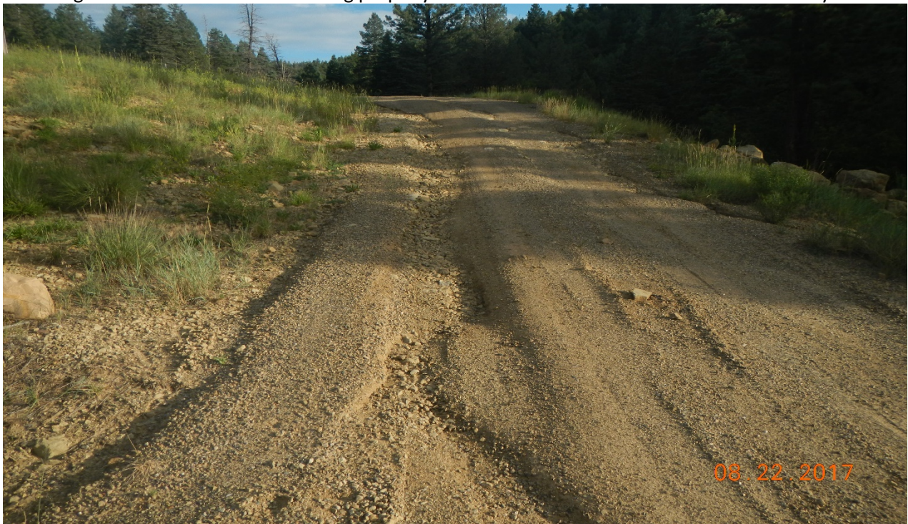
photo 2: Facing northwest at the access road. Signs of erosion indicates stormwater is flowing down towards the main road. A culvert may be needed at this point.
