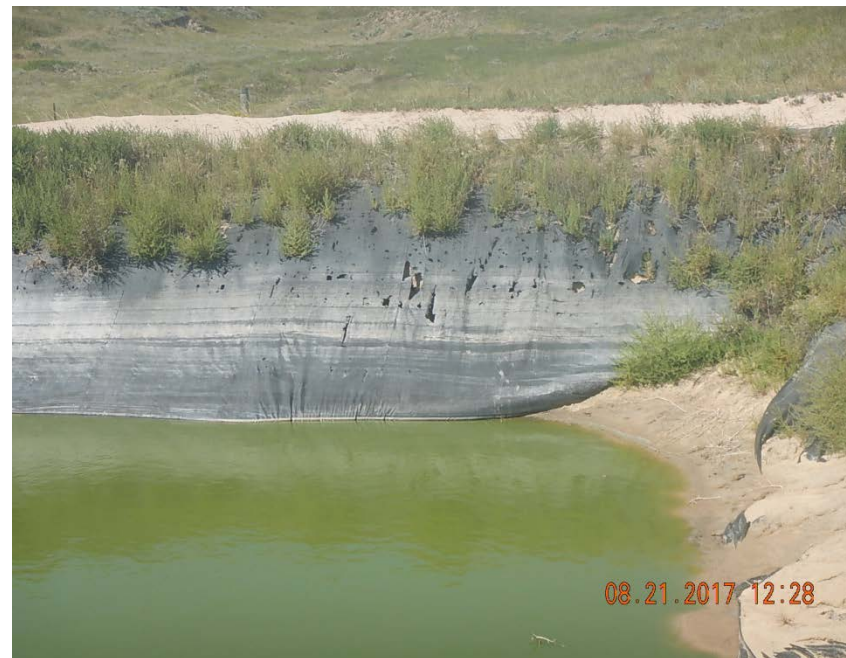
Photo 8: Tears in liner, vegetation in liner
