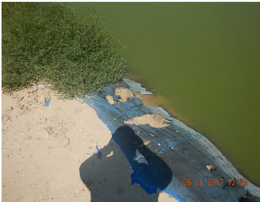
Photo 5: Tear in liner
