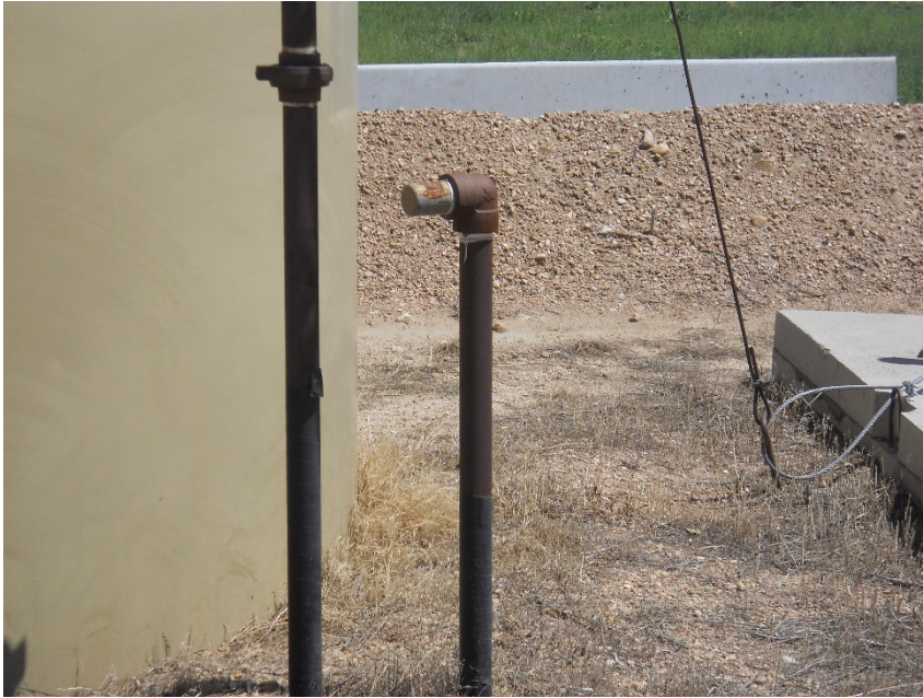
Unused/unmarked 2" riser southwest side of crude tank
