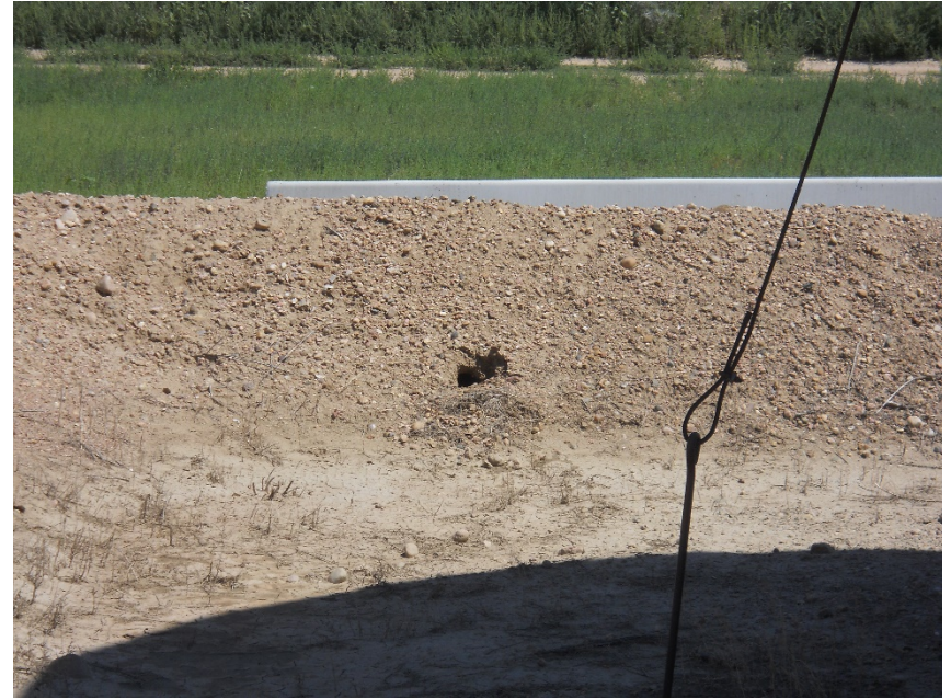
Animal burrow inside of tank berm northeast side
