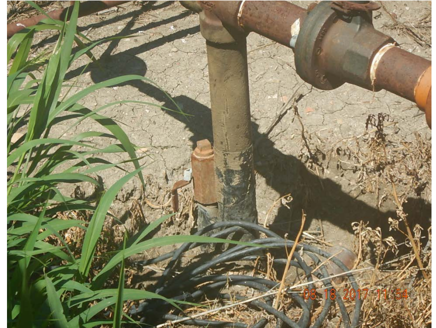
Photo 2: 1-1" riser at wellhead
