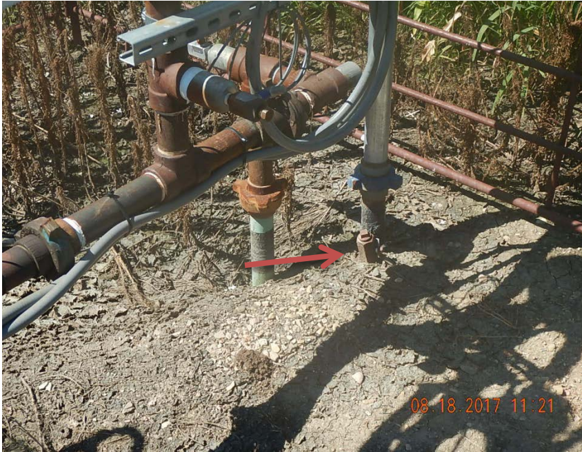
Photo 3: 1" riser at wellhead
