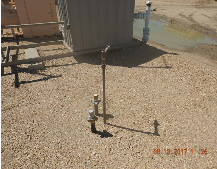
Photo 5: 2-2", 1-1" risers at meter run
