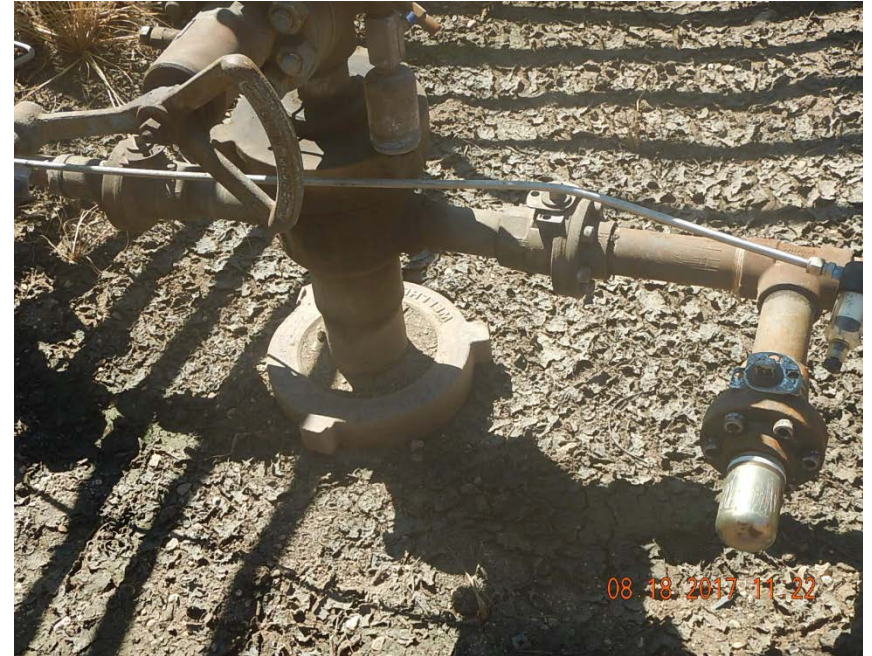
Photo 4: No bradenhead at surface of 4-2-32
