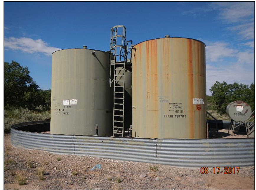
Photo 4. Condensate tanks labeled OUT OF SERVICE.
