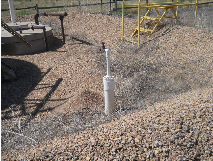
Unused/unmarked riser inside of tank berm on northwest corner
