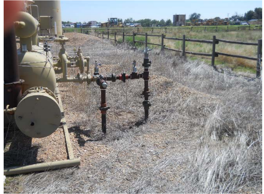
Flowline at separator is still in place. Dead weeds on south side of location pose a fire risk. Needs to be controlled.
