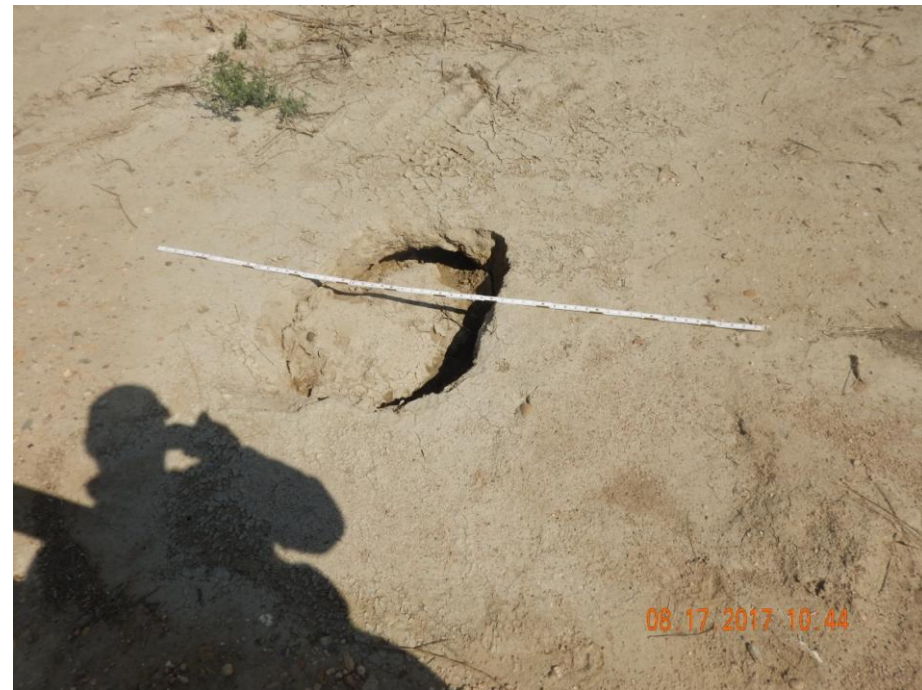
Photo 3: Photo taken from the battery location. Inspection doc. #682502204 required operator to repair subsidence. Photo shows subsidence remains and appear to have degraded further. This needs to be repaired. 6 foot measuring stick for reference.
