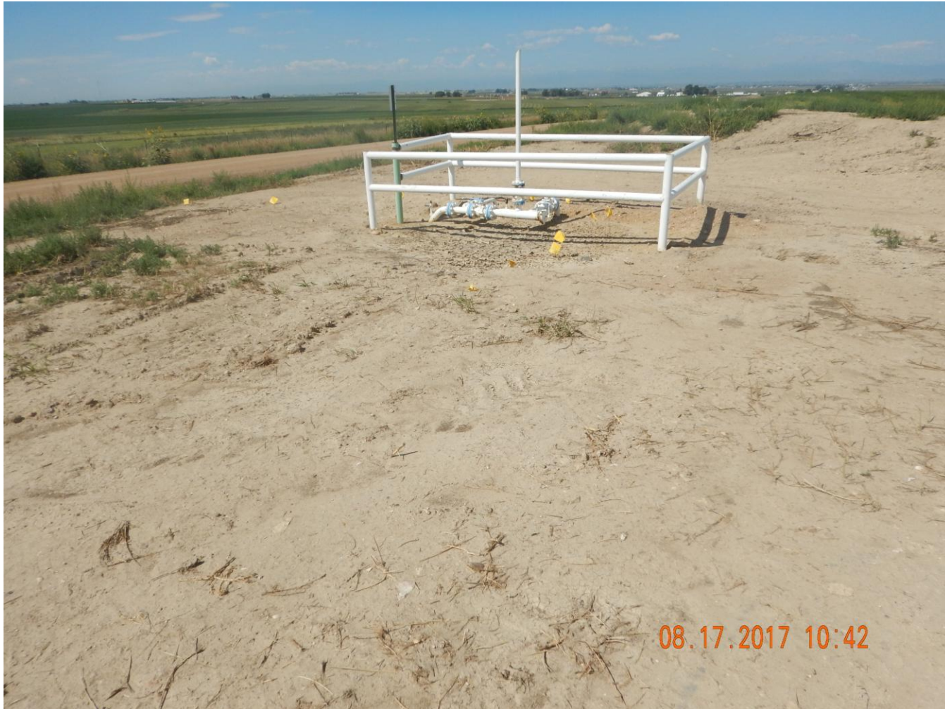
Photo 1: Photo taken from the battery location, facing west. Photo shows risers have been removed per CA.
