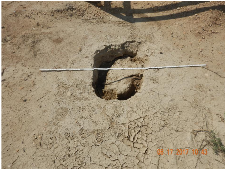
Photo 2: Photo taken from the battery location. Inspection doc. #682502204 required operator to repair subsidence. Photo shows subsidence remains and appear to have degraded further. This needs to be repaired. 6 foot measuring stick for reference.
