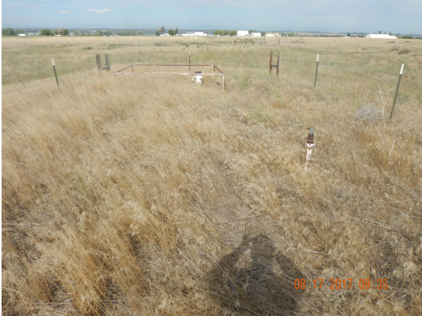
Photo 1: Photo taken from the east end of the location, facing west. Inspection Doc. # 682502155 required operator to remove risers from the location. Photo shows pipe risers still remain.
