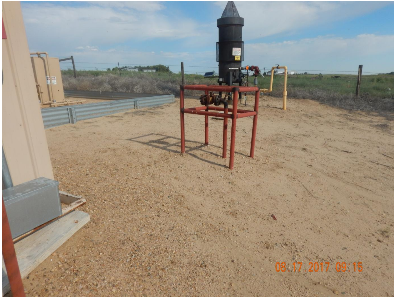
Photo 1: Photo taken north of the battery facility, south of the well. Inspection doc. #682502147 required operator to remove riser. Photo shows riser still remains.
