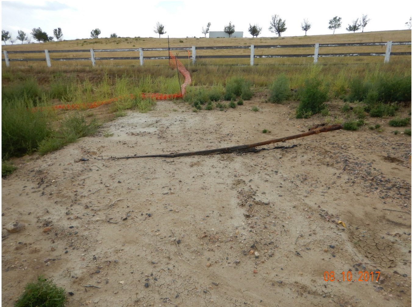
Figure 5 - Rusted, abandoned 2" steel flowline daylighting west of former excavation.
