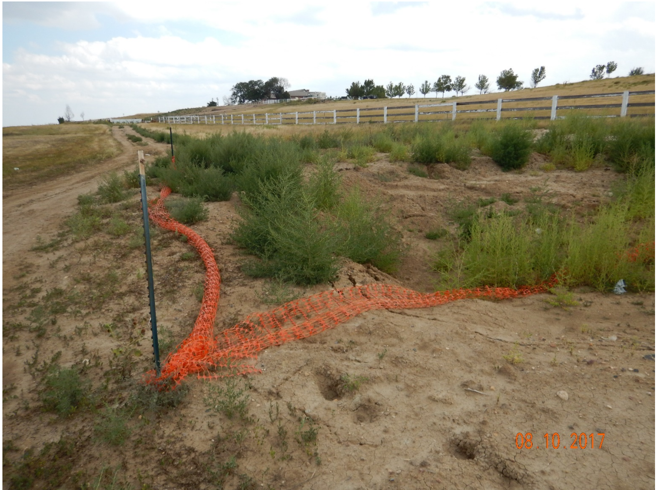
Figure 3 - View of backfilled excavation associated with Remediation Project #10065 from NW corner. Note: abundance of weeds and subsidence inside of damaged safety fence.
