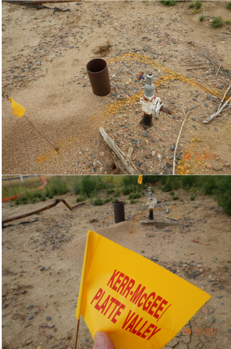
Figure 6 - 2" steel flowline riser and ~6" pipe riser on west side of former excavation. Yellow flags and markings suggest that the flowline is operated by Kerr-McGee/Platte Valley.
