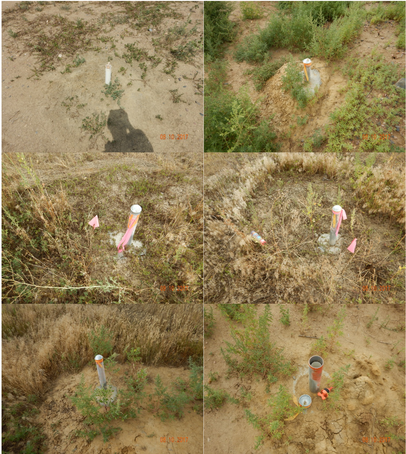
Figure 11 - Assorted pictures of monitoring wells installed at location under Remediation Project #10065.
