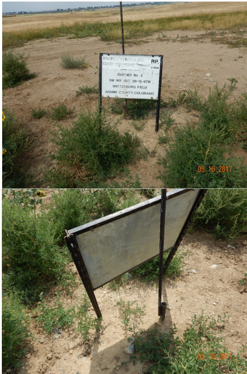
Figure 1 - Well sign at former well location is supported by buried polished rod.
