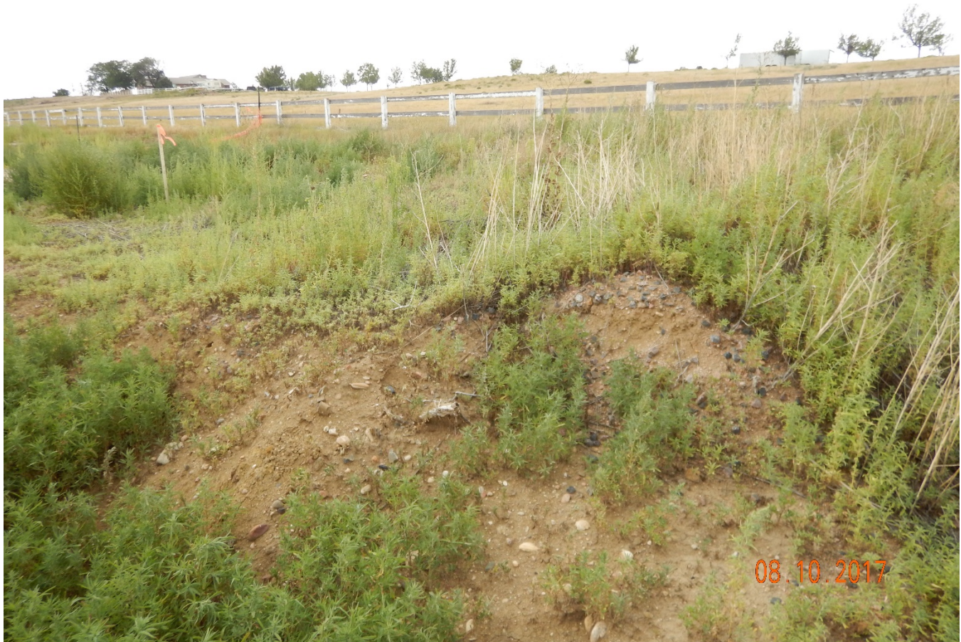
Figure 7 - Cross-sectional view of former vertical treater berm that remains on location (west of former excavation). Grade has not been restored to preexisting conditions. Uncontrolled weeds and gravel remain on-site.
