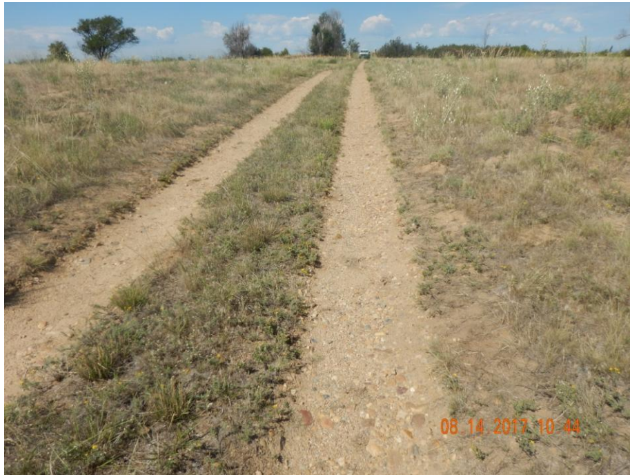
Photo 5: Photo taken from the access road, facing west. Photo shows access road has not been reclaimed per CA's from inspection doc. #682502088
