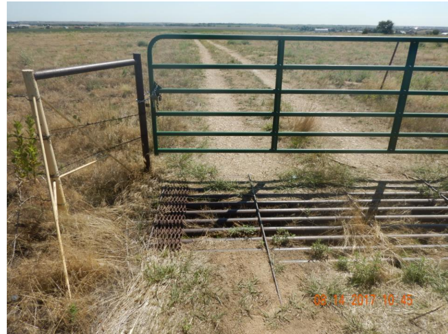
Photo 6: Photo taken from the access road, facing east. Photo shows cattle guard, access road and gate have not been reclaimed per CA's from inspection doc. #682502088
