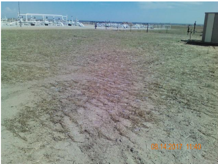
Photo 1: Photo taken from the southwest corner of the tank battery location, facing northeast. Photo shows tank battery location appears to have been seeded, then crimped with straw to stabilize the soil.
