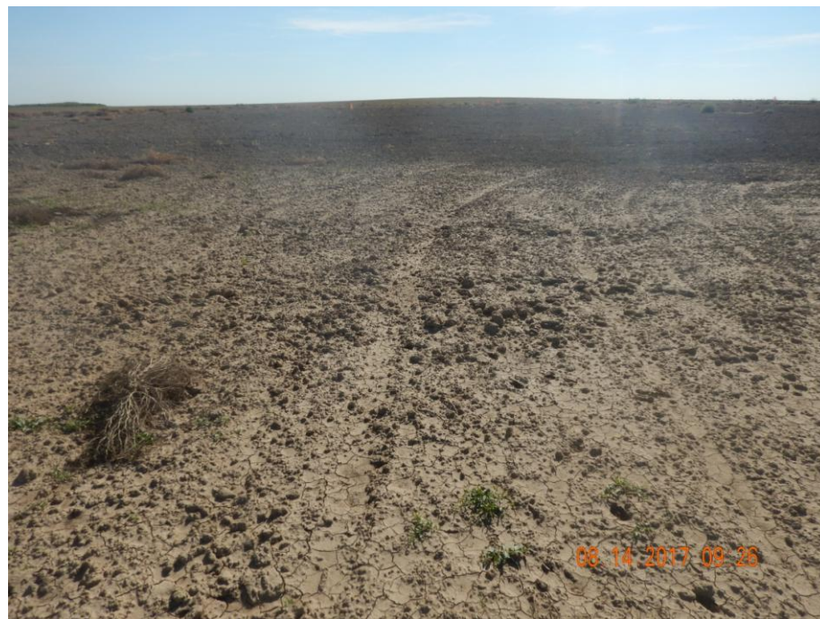
Photo 2: Photo taken from the west end of the location, facing east. Photo shows no additional BMPs have been implemented and used in conjunction with surface roughening per CA's from inspection doc. #682502162
