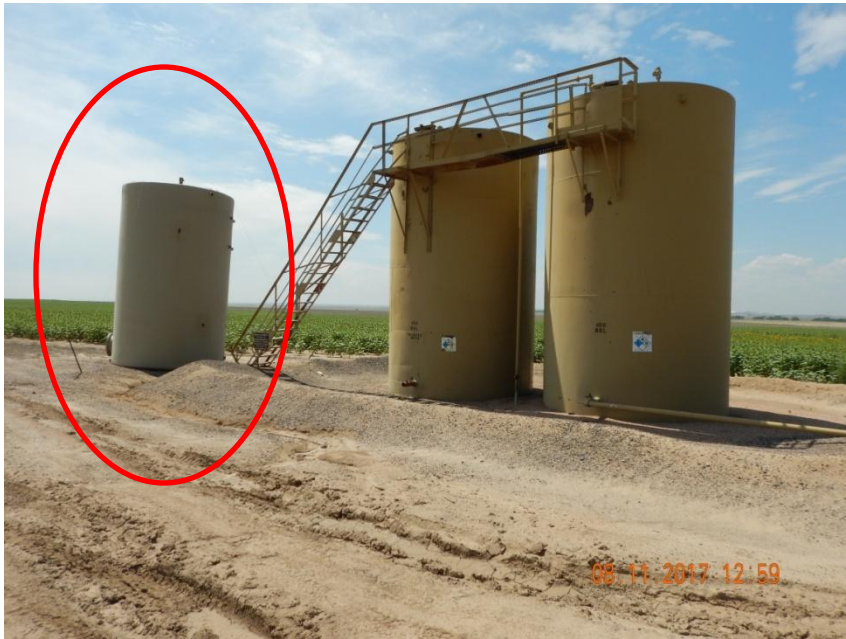
Photo 3. Photo of the tank battery location, facing Southwest. Appears an unused tank is being stored at location and needs to be removed within 90 days of this inspection.
