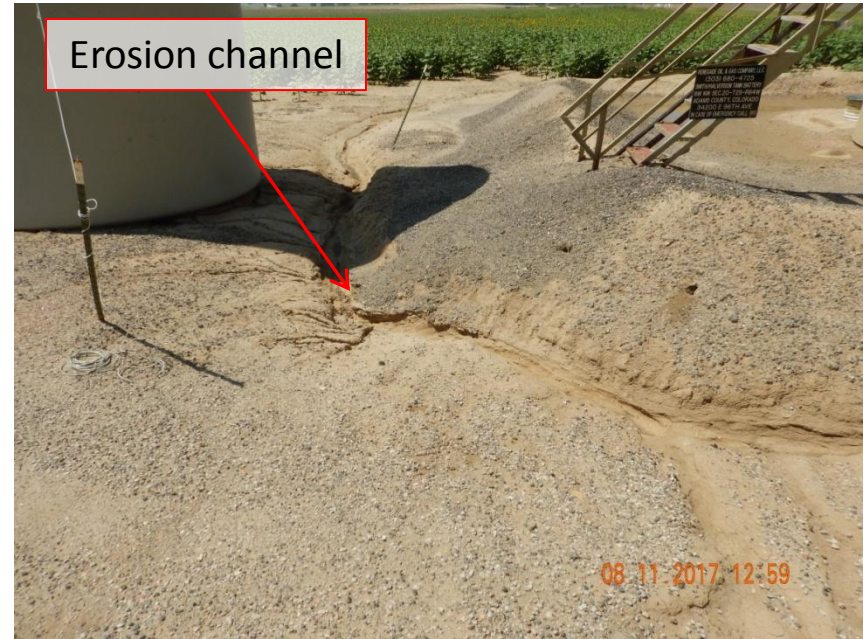
Photo 4. Photo taken from the eastern tank battery location, facing West. Gully erosion forming at location that is contributing to sediment discharge off location.
