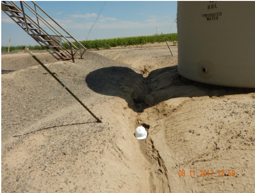
Photo 5. Photo taken from the western tank battery location, facing East. Gully erosion forming at location this is contributing to sediment discharge off location.
