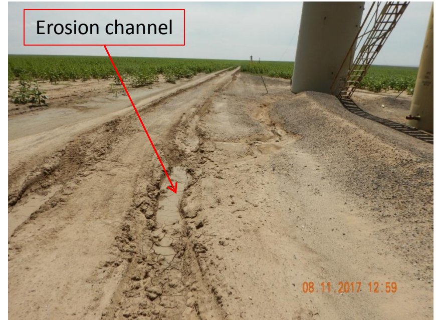
Photo 2. Photo taken from the entrance of the tank battery location, facing South. Stormwater erosion evident as an erosion channel funnels around the northern battery location and continues off location into the adjacent cropland.
