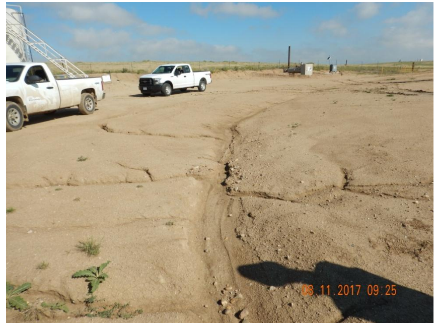
Photo 2. Photo taken from the southeastern well location, facing Northwest. Rill/gully erosion throughout the location that is causing sediment discharge off location.
