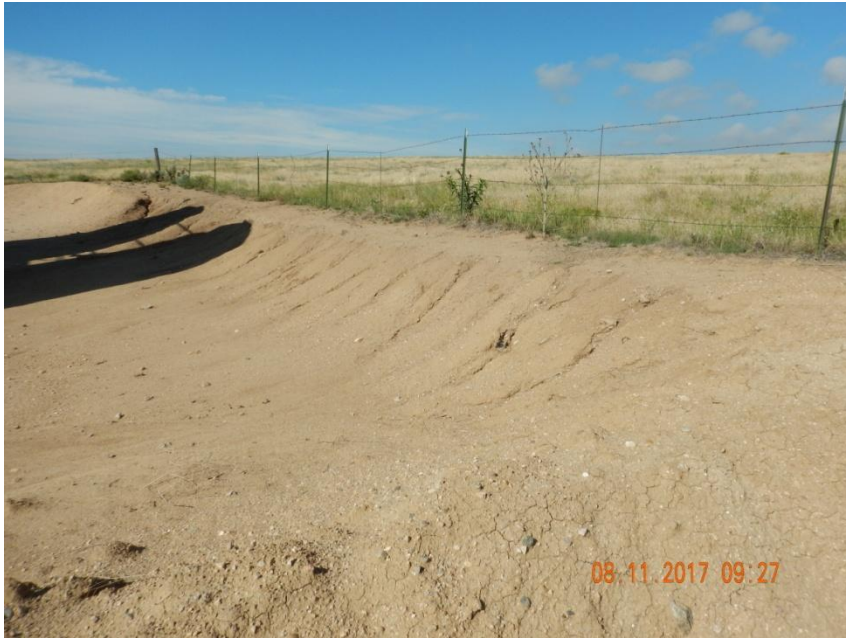
Photo 5. Photo taken from the western location, facing Southwest. Rill erosion occurring throughout the cut slope contributing to sediment discharge off location. Cut slope needs to be stabilized to prevent erosion and stabilize the production area.
