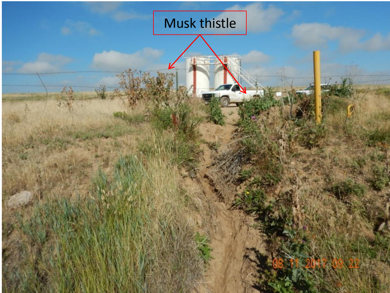
Photo 3. Photo taken from the discharge point, facing West. Gully erosion occurring this is causing sediment discharge off location. Also, a List B Colorado Noxious weed, Musk thistle, shown in this photo and was observed throughout the well location and access road.
