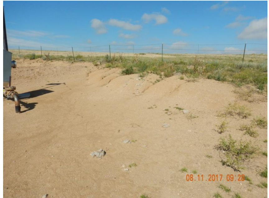
Photo 6. Photo taken from the northwestern location, facing Southwest. Rill erosion occurring throughout the cut slope contributing to sediment discharge off location. Cut slope needs to be stabilized to prevent erosion and stabilize the production area.
