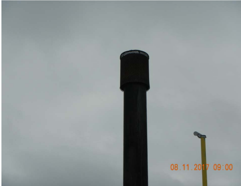
Installed separator bird screen
