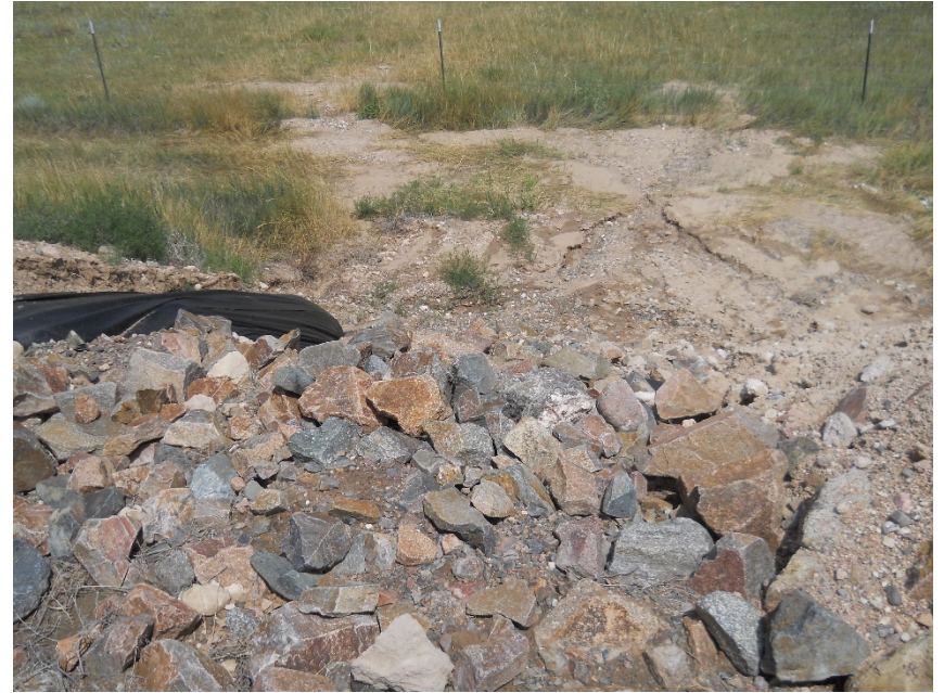
Erosion at discharge run down on north side of battery
