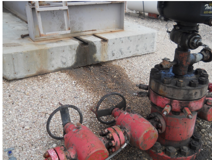
Stained soil at wellhead and pump jack skid
