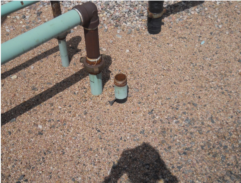
Unused/unmarked 3" riser on east side of north crude tank
