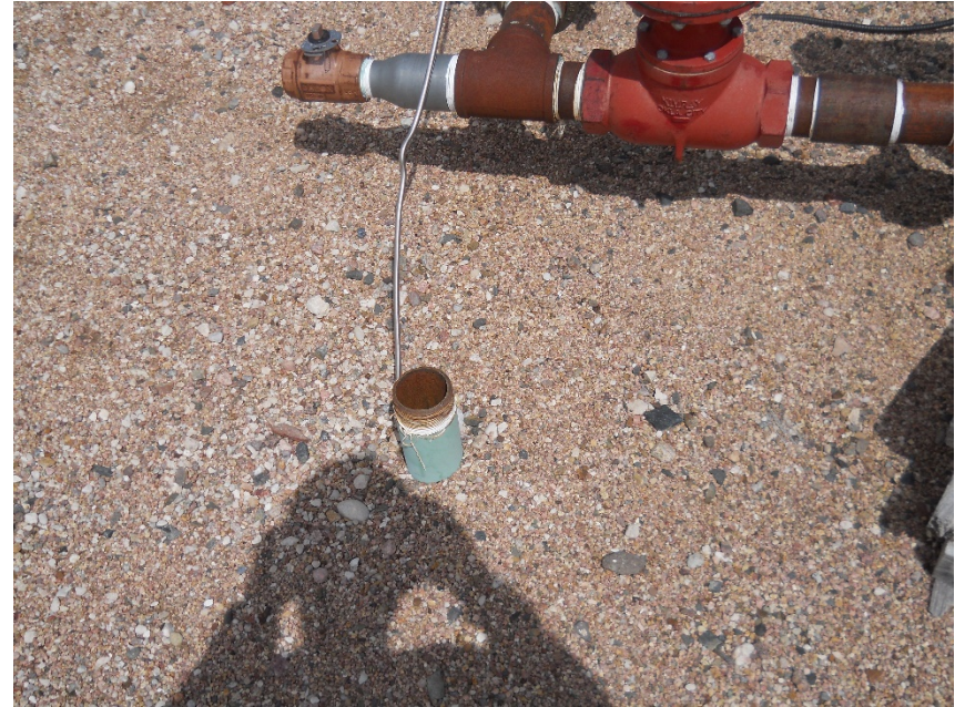
Unused/unmarked 3" riser on south side of ECD
