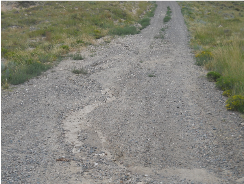
Erosion on lease road hill looking south
